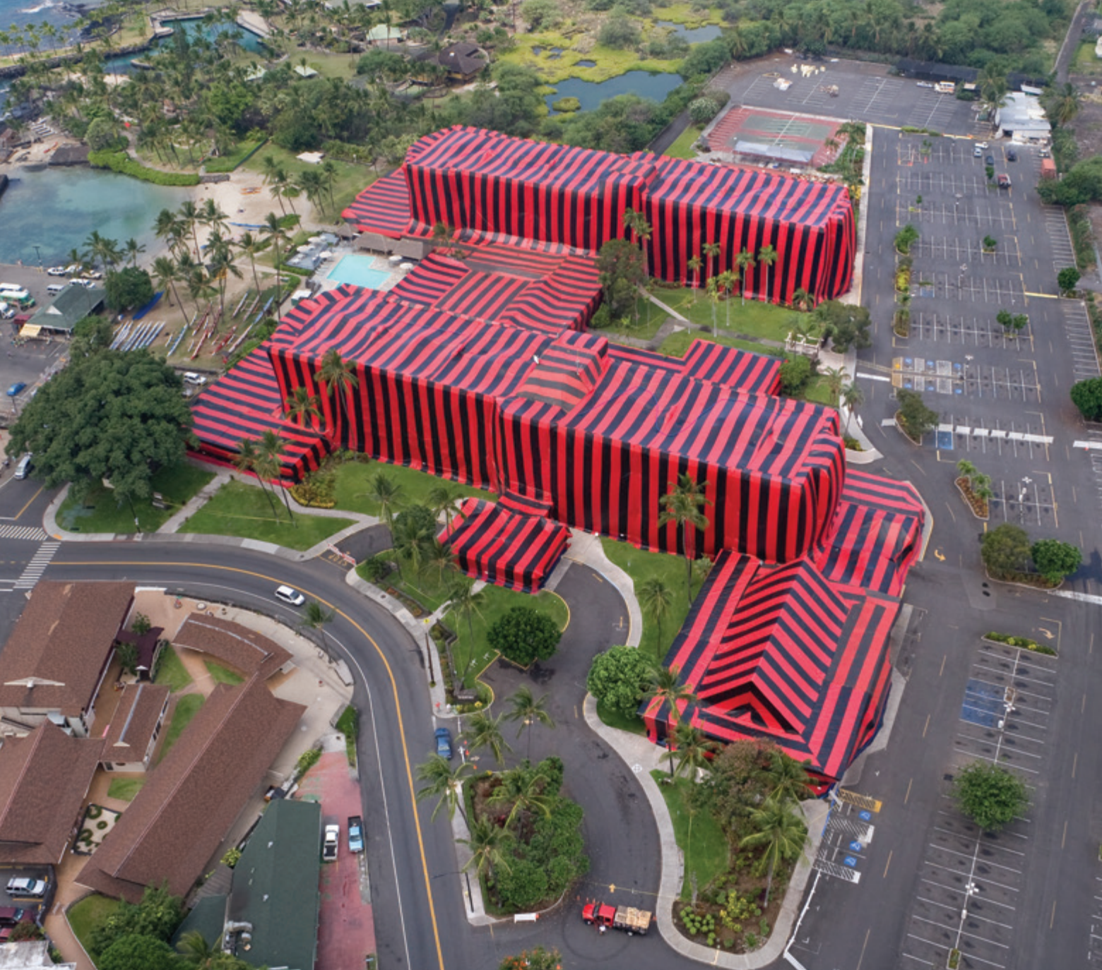
Bedbug infestation was so bad at the King Kamehameha Hotel in Kona, it required tenting the entire structure
