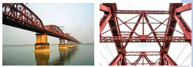
Photos 11-12. Hardinge Bridge with High Tension Transmission Line. The repair of Pier 2 by confining is also visible in left figure. Top chord bracing of the repaired span 12 is seen in the left with electric transmission lines both upstream and down stream are seen. Images by: A.F.M.S. Amin
