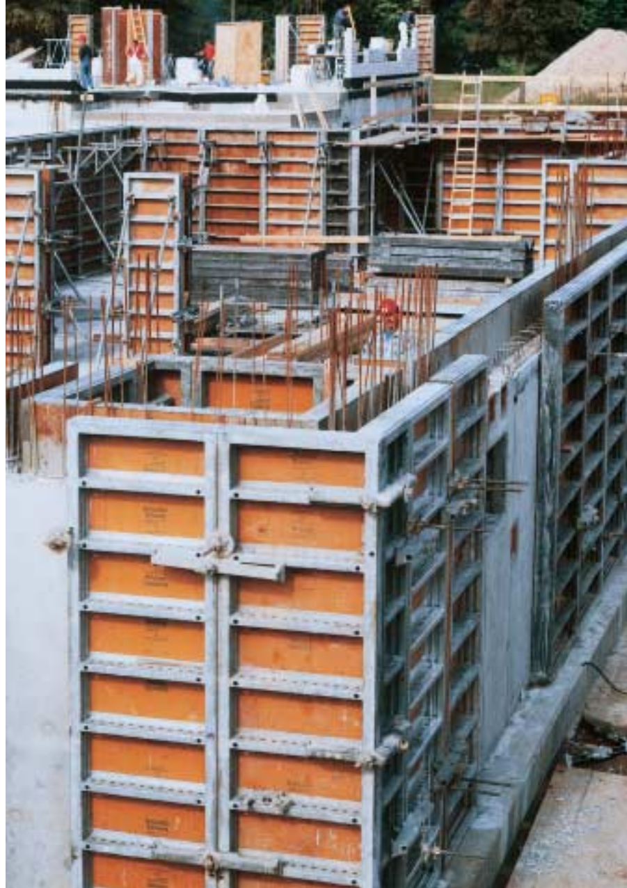
The outer corner is designed for the full amount of concrete pressure. For wall thicknesses of 2.70 m, only three outer corner clamps are needed!
