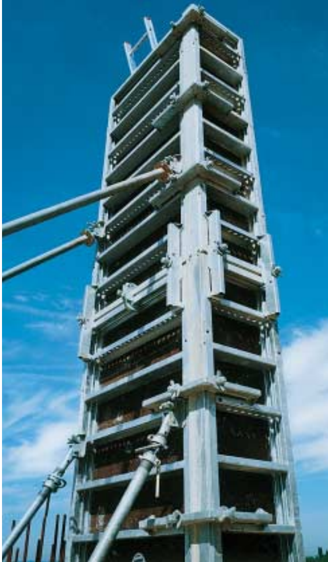
The outer corner clamp is also the ideal connection means for column formwork.
