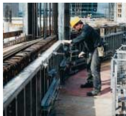
MANTO waler for length compensations of up to 30 cm and for the stopend. Can also be used with acute- and obtuse-angled corners.
