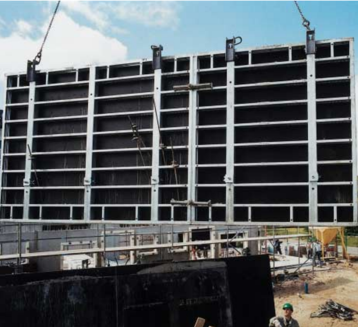
Tension/compression brace at the head of the formwork Picture of the system
