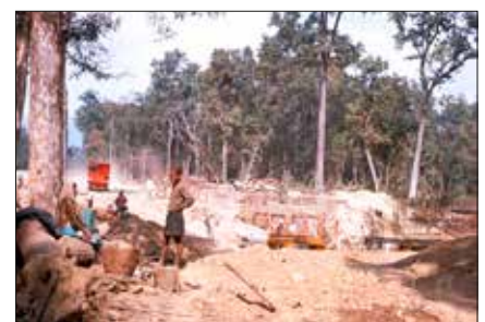
Building works on the East-West Highway across Nepal 1968
