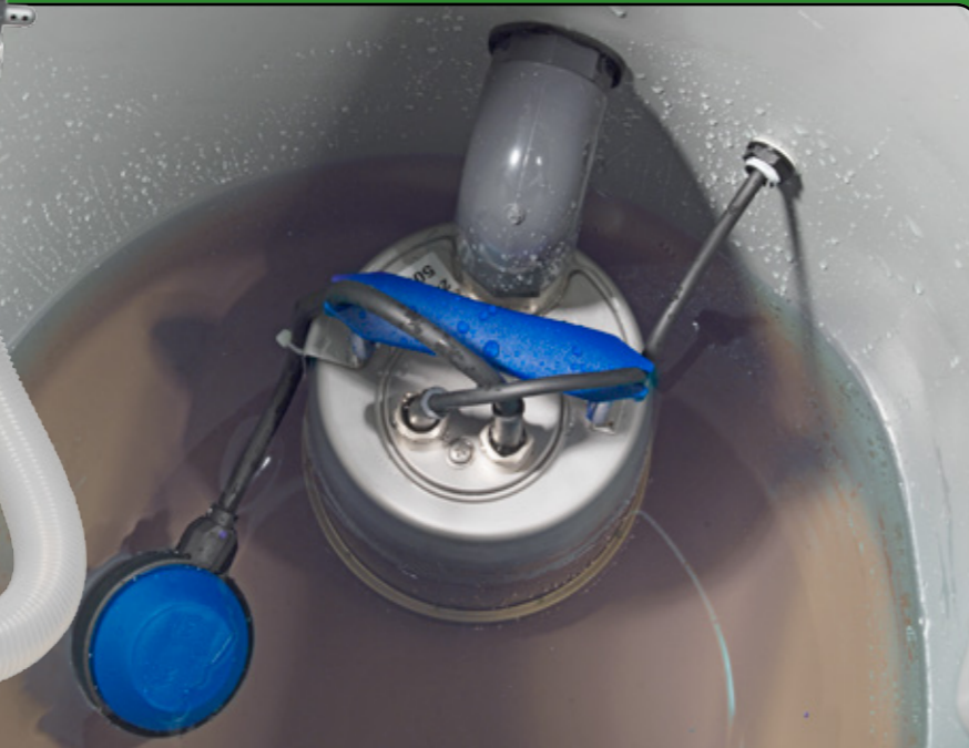
AP submersible pump system
