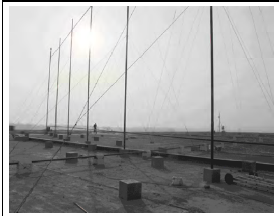
Fig. 7: Realized Wire Fence, Numerical Design
