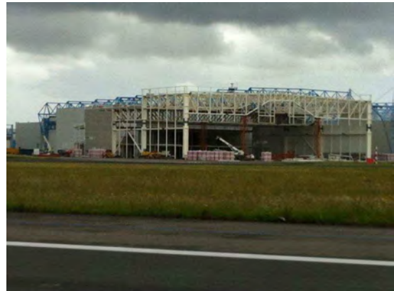
Figure 12. Start of first skin erection of east facade
