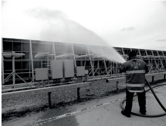
Figure 6. Water Saturation Test of Localizer Antenna and Blast Fence
