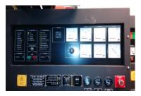
The system was to have four generators independently backing up separate mains on each of the four blocks to work as 'no break return' operation along with individual G59/3 protection on each.
