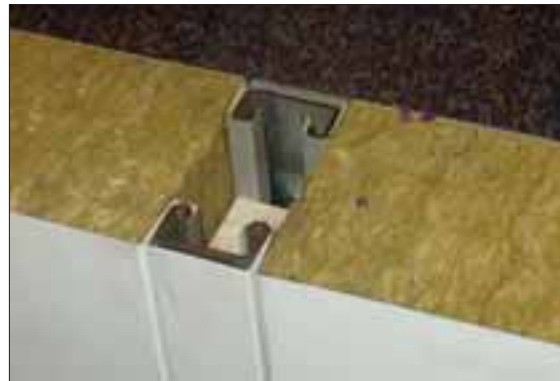
Figure 17: Insulated core panels – internal panel
