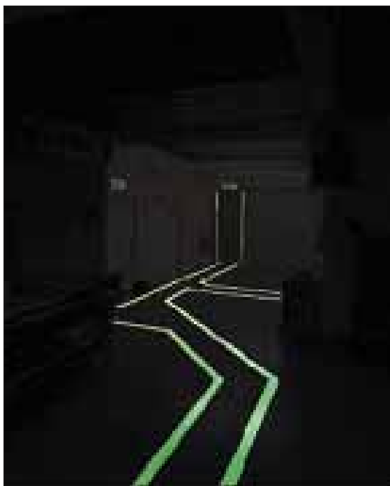
Figure 52: A 'way-guidance' system
