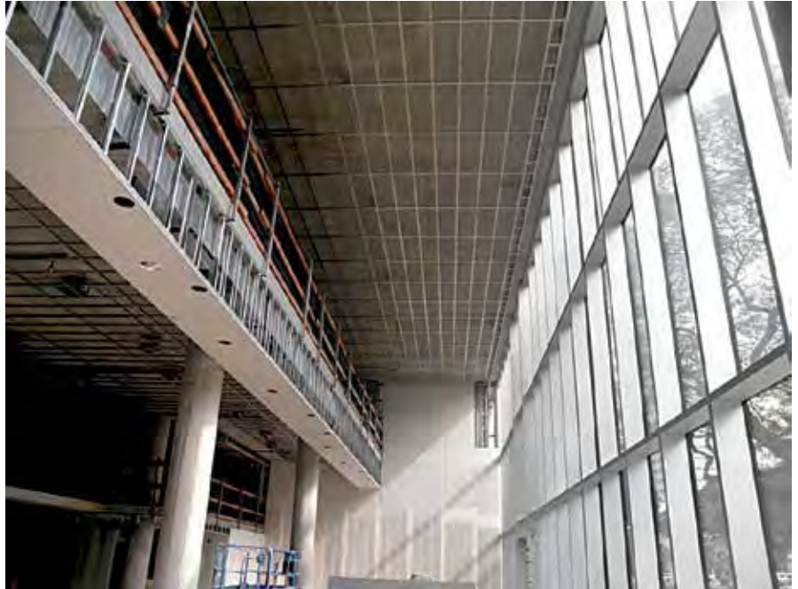
Build-out of Velocity's high ceiling frame for Audi PHOTO COURTESY UNLIMITED CONSTRUCTION SERVICES INC.
