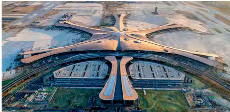
An aerial view of Beijing Daxing International Airport under construction.
