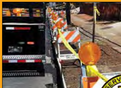
Temporary Traffic Control
