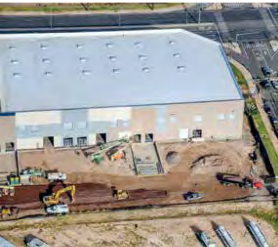
View of work in the loading dock area
