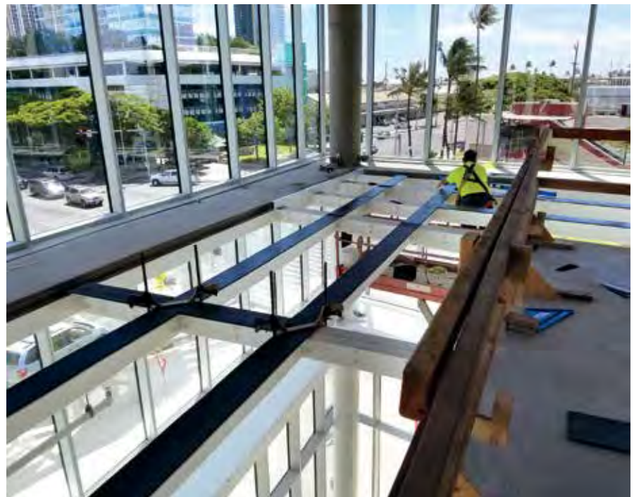
Installing steel frames for Velocity's third-level glass floor PHOTO COURTESY AHL
