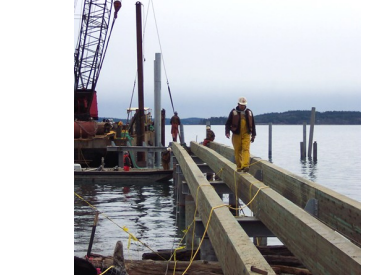
Recent construction photos.
