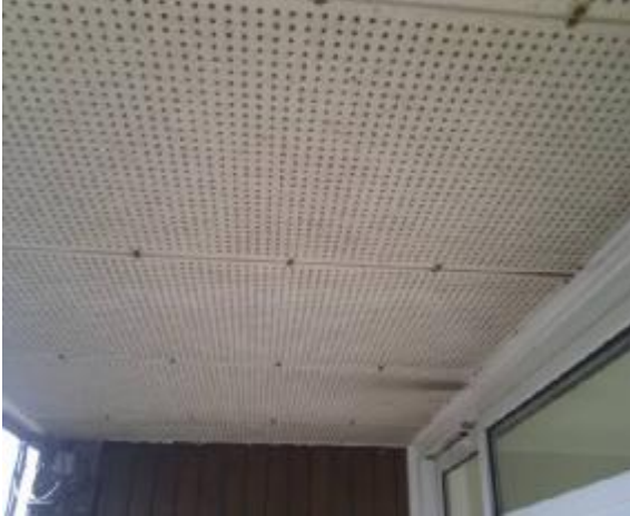
Perforated AIB Ceiling panels to 44 Balconies
