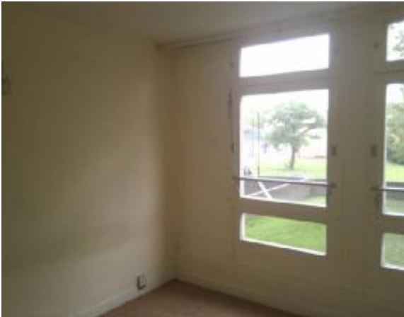
AIB Window Panels to 88 dwellings
