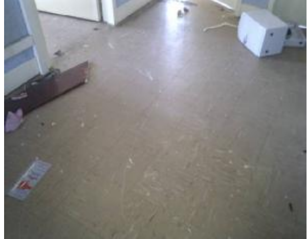
Thermo-plastic floor tiles to 88 No' dwellings
