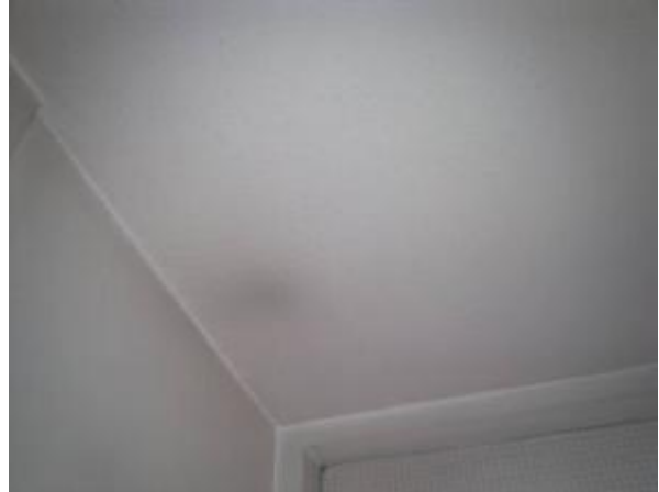
Textured Coatings to 4400M 2 of ceilings
