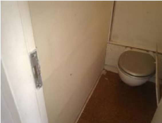
AIB Duct Panel removal to 88 Bathrooms and WCs
