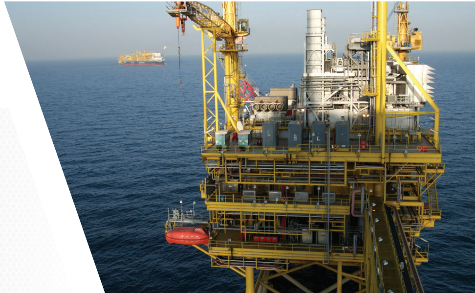
Real-time drilling capabilities with Harris CapRock's VSAT solutions
