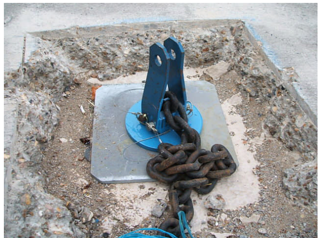
Existing holes in the footpath are used for chain suspension.
