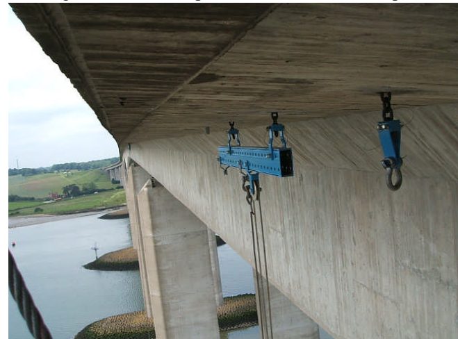
Existing holes in the footpath are used for chain suspension.
