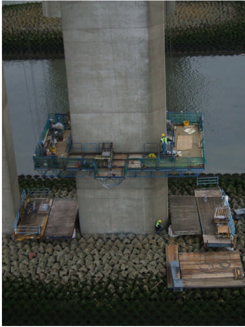
With the platform constructed & examined it travels at 3M min': Main platform in place at high level ready for work.
