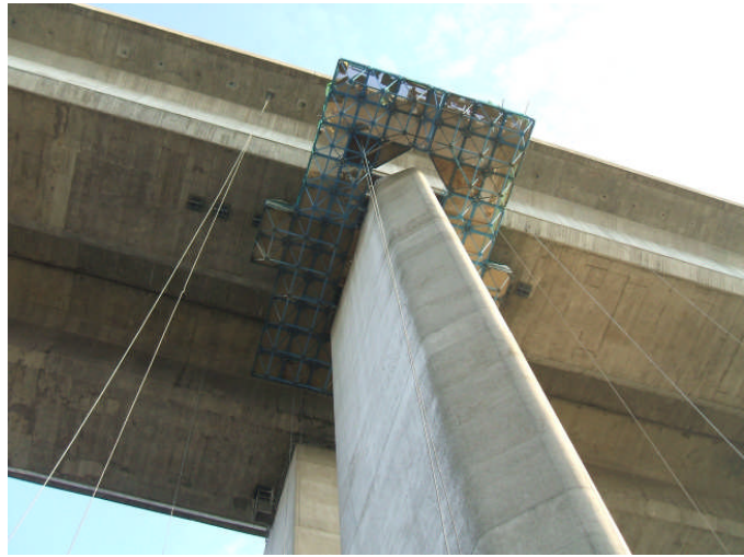
With the platform constructed & examined it travels at 3M min': Main platform in place at high level ready for work.
