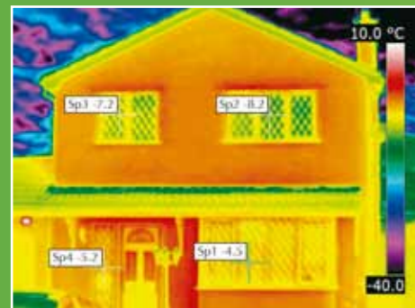
Red areas have been eliminated after fitting energy efficient VEKA windows.
