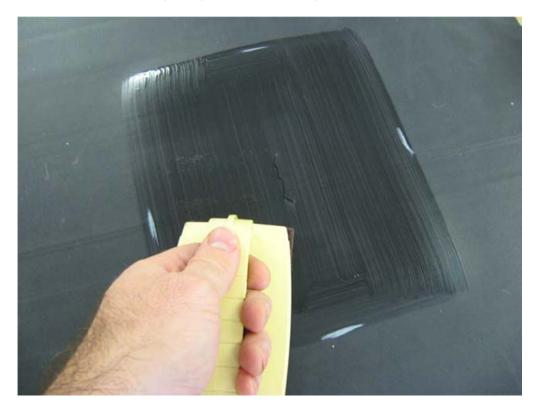
Cuts and punctures in the membrane should be repaired with cured cover strip. Cut out a piece of cover strip tape or FormFlash 75mm larger than the puncture and round off the corners. Remove the backing paper and apply over the puncture. Roll with the silicon hand roller.
