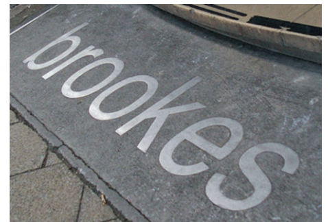
Stainless steel letters cut from sheet metal. Mounted into paving.
