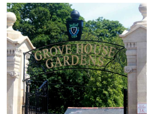
Letters and crest cast in polyurethane. Mounted onto a custom mad iron arch.
