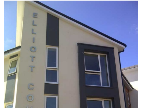
Stainless Steel built up letters Rear mounted studs are cemented into pre drilled wholes in the substrate
