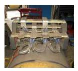
Fig 1. Terminal box assembly dirt build-up.
