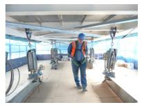
TOWER BRIDGE is possibly the most iconic and internationally recognised bridge in the world; when it required a facelift ALPS were asked to supply a bespoke suspended access solution to enable preparation and painting works to be carried out to the underside of the upper walkways. Due to road closure time restraints conventional scaffolding was not an option.
