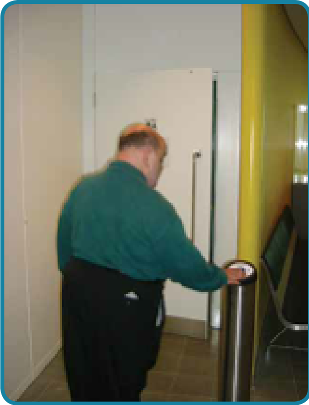
The automatic door to the CP toilet at City Hall, London. The push pad should be 750-1000mm above floor level and set back 1400mm from the leading edge of the door when open
