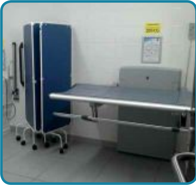
A wall-mounted changing bench at Cherwell Valley Moto Services. It is height adjustable, with maximum-load capacity and instructions clearly on display
