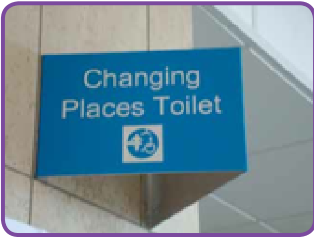
Double-sided overhead signs are visible from different directions. In this example from Middlesbrough Bus Station, the logo is used with the words 'Changing Places Toilet' in clear print and in title case, which is easier to read
