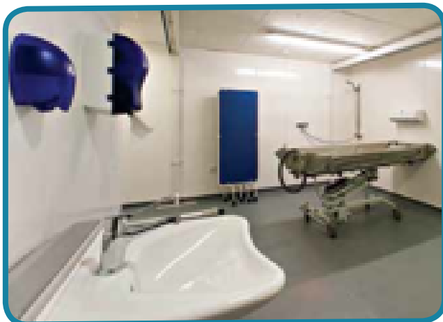
Height-adjustable washbasin with flat sides to rest arms and a lever mixer tap at Warminster Civic Centre
