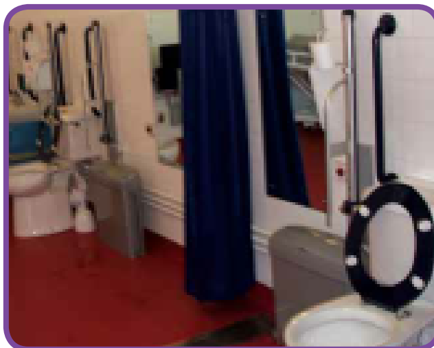
Keighley Leisure Centre's 23 sq m facilities are large enough to include two peninsular layout WCs with a privacy screen, enabling more efficient use by a visiting group
