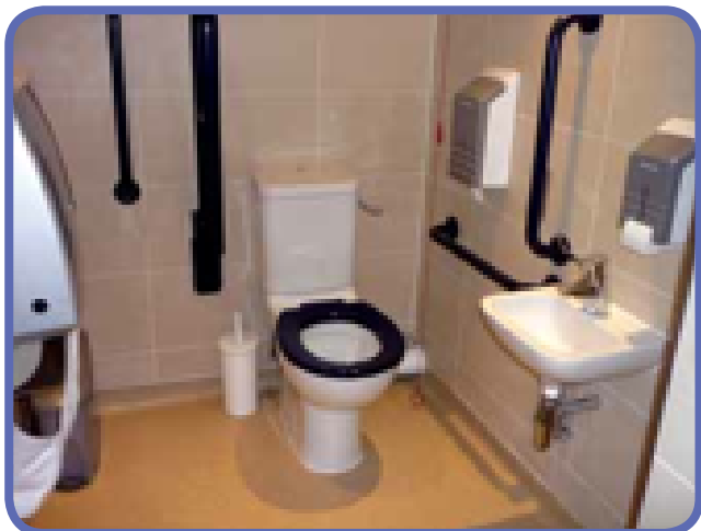
Standard accessible corner WC for independent use: minimum 1.5m by 2.2m in size, no equipment or space to change an adult or for assistants
