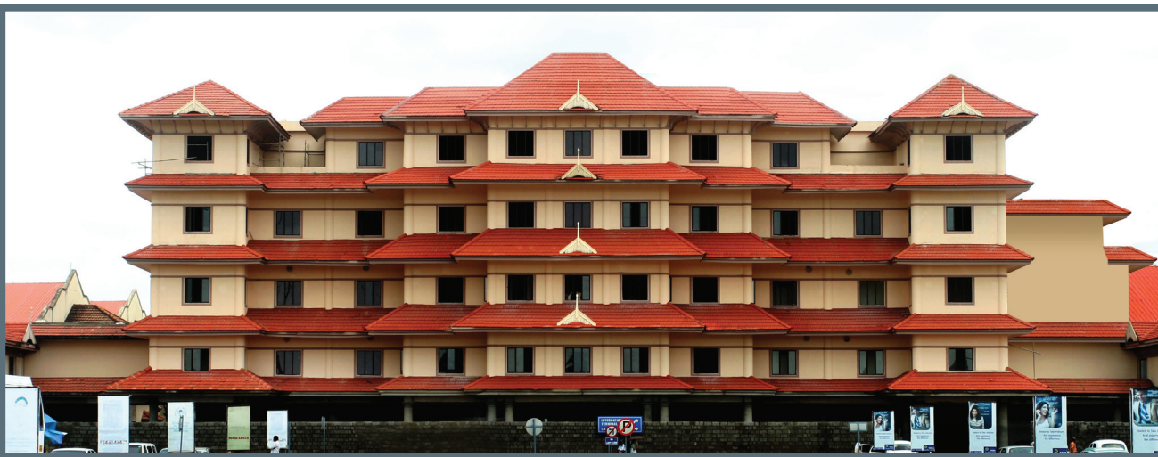
Cochin International Airport, Nedumbassery
