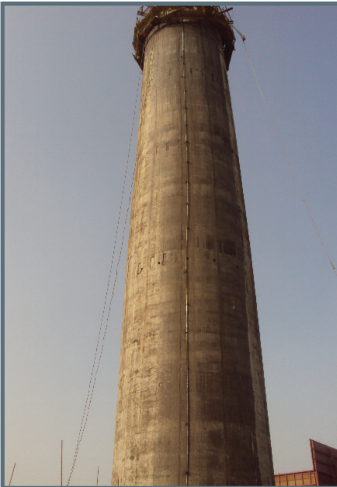
JSW, Bellary – Chimney
