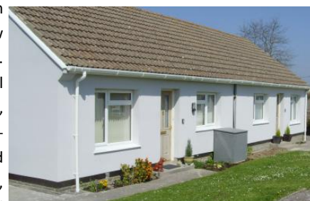
Above: Insulation works, Fivehead (Completed)
