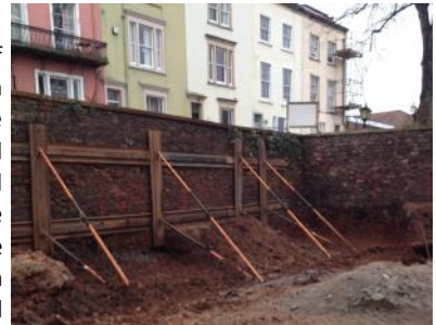
Above: Clifton Park, Bristol (Retaining wall works)
