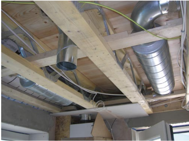
Figure 14. M&E installation integrated through the webs of the eco-joist suspended floors.
