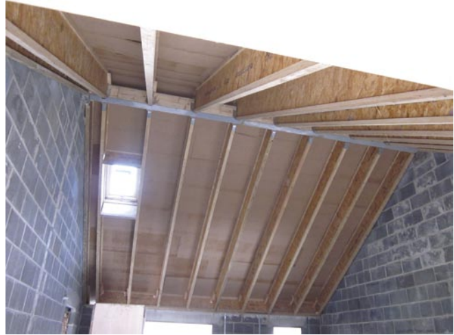
Figure 5. Below: the finished open cathedral ceiling to an upstairs flat with mezzanine bed platform.
