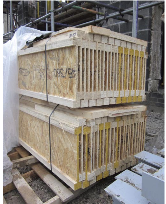
Fig 3. Picture of the 350mm JJI roof rafters delivered to site ready for erection.
