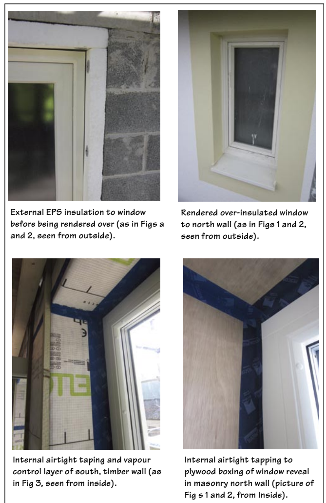
Fig 7. Various shots of airtight tapes and exterior view of over-insulated window.
