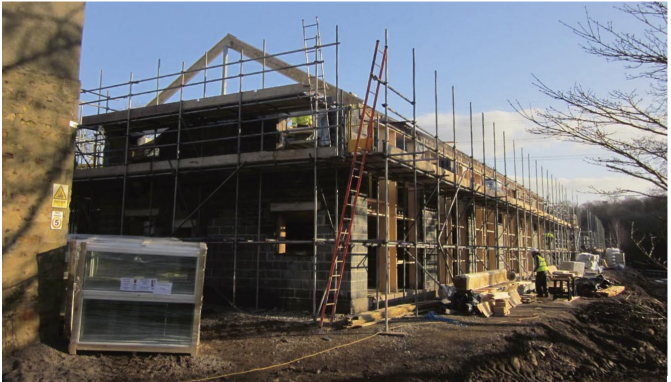
Above: showing the project well underway with many of the masonry structures completed ready for roofing. Below: the site layout.
