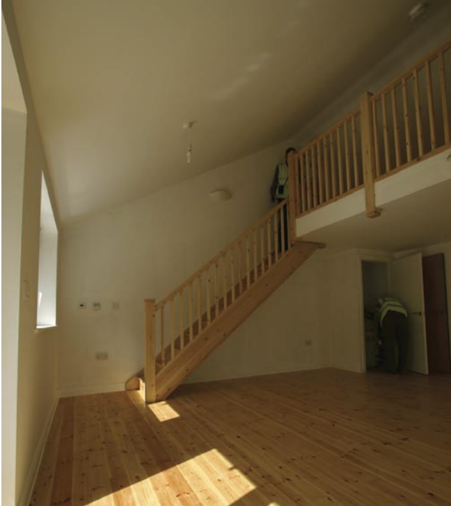
Figure 5. Below: the finished open cathedral ceiling to an upstairs flat with mezzanine bed platform.
