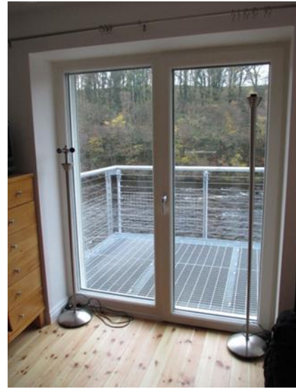
Figure 3: Windows locks and handles were fiddly with no fine control adjustment
