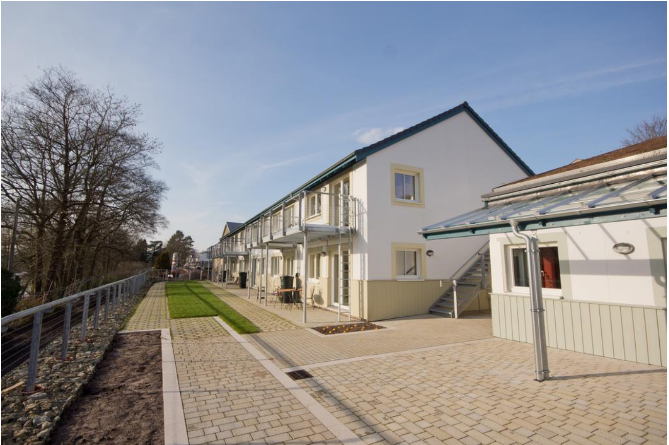
Picture 2: Typical View of the completed houses & the Common House Community Terrace
