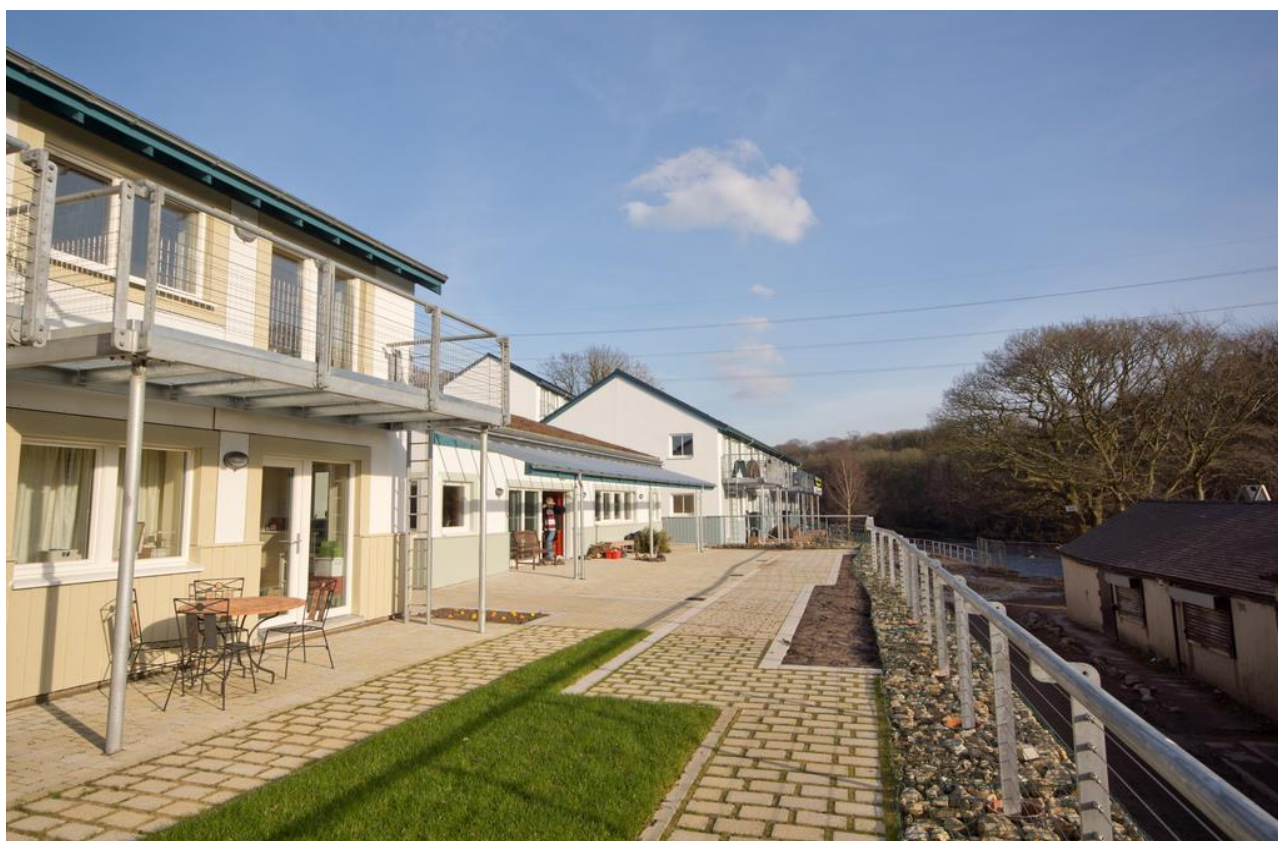
Picture1: Typical view of the completed Passive houses & the Common House Community Terrace
