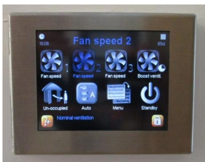
Figure 2: The MVHR programmer was easy to understand but does not alert the occupant to blocked filters.
