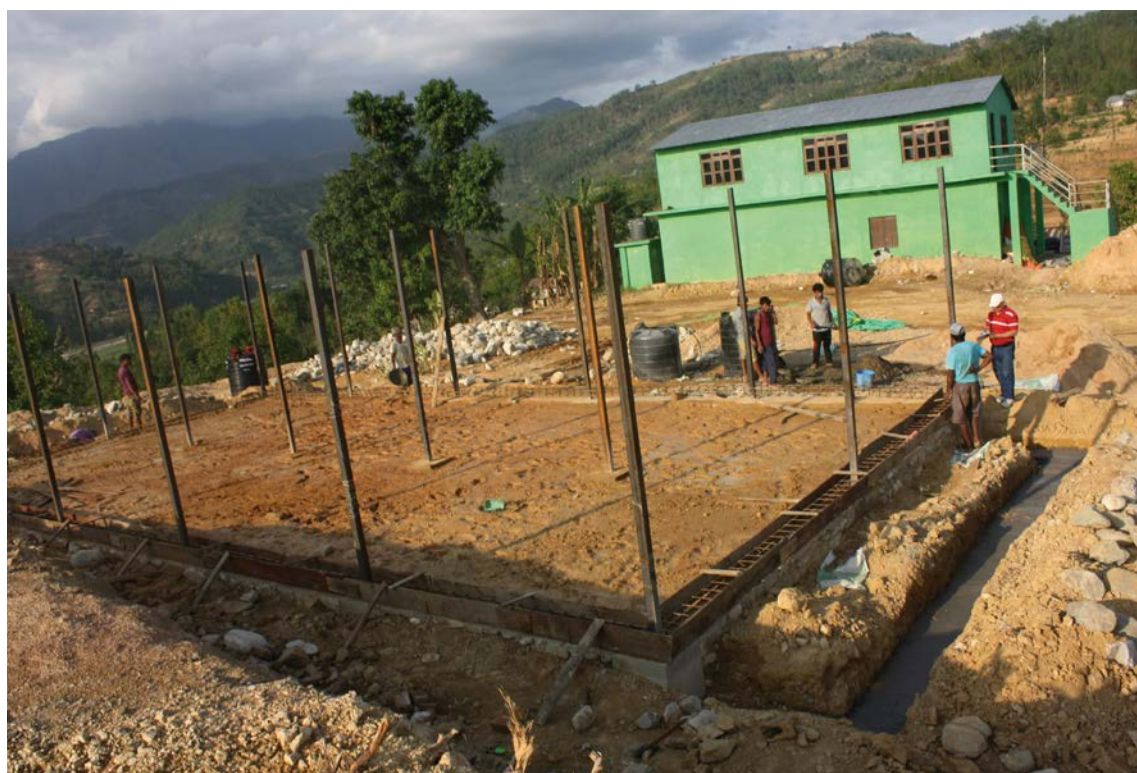
Building under way in Makwanpur
