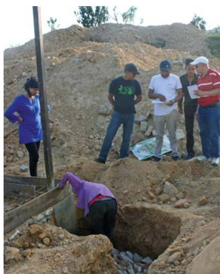
Preparing the construction site
