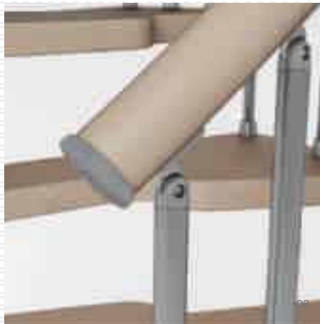
03 _ Detail of handrail end cap.
