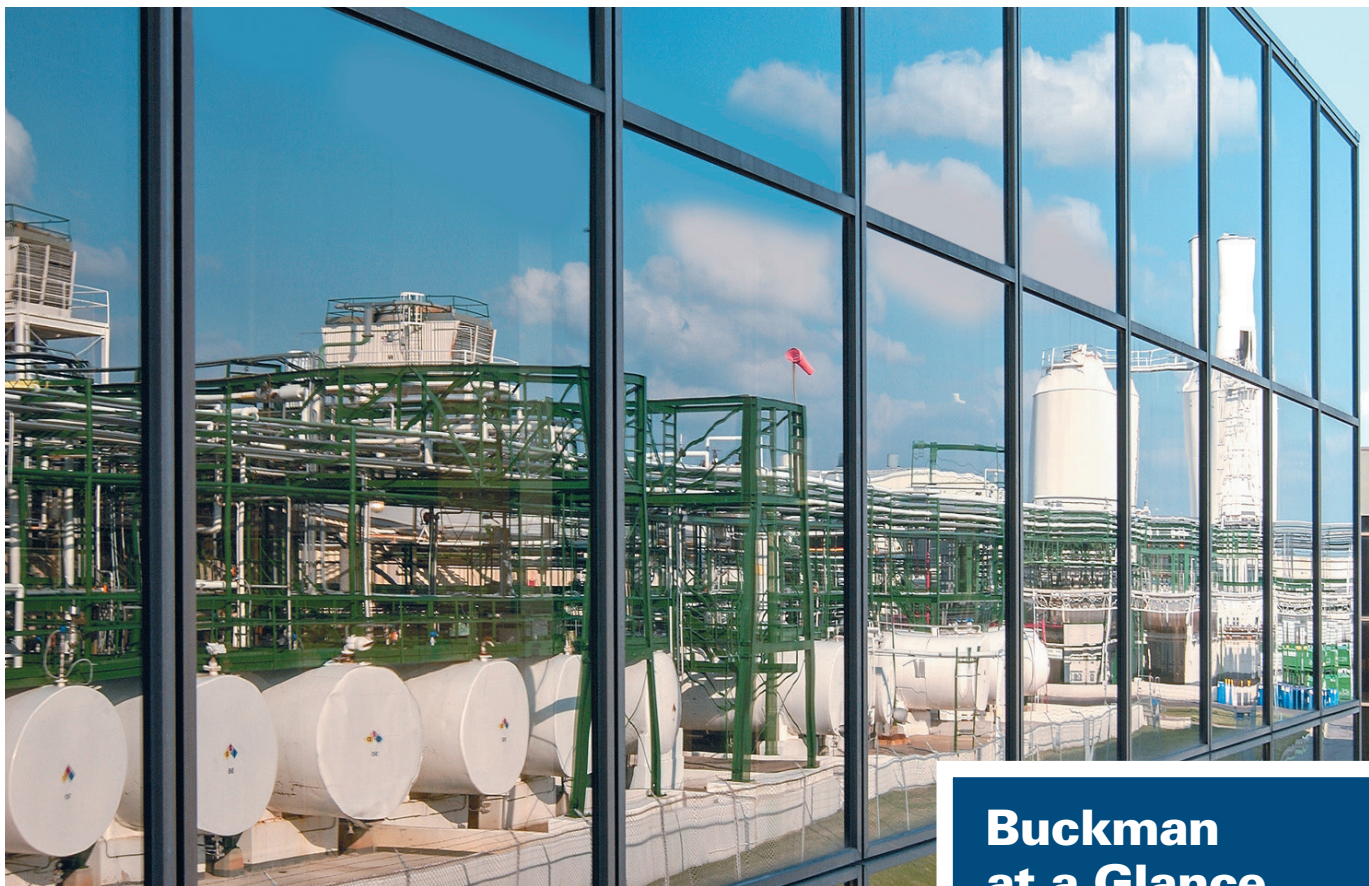
Buckman's global headquarters in Memphis, showing a reflection of its adjacent manufacturing facility.
