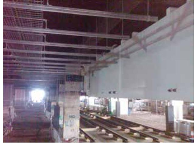
A purpose built track was then constructed to run the full length of the station to spread the load of each module equally across the concourse, reducing direct load to the concrete deck.
