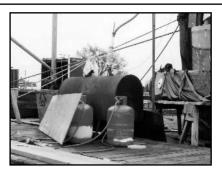
The boiler used to steam the planks so that they would bend in to shape on the hull.
