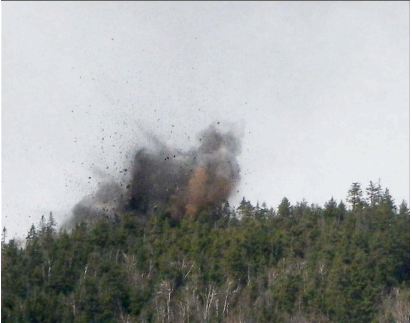
Uncontrolled Blasting, Lowell Mountain, Vermont
