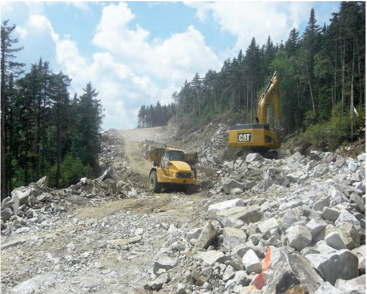
Road to Mt. Kelsey After Blasting
