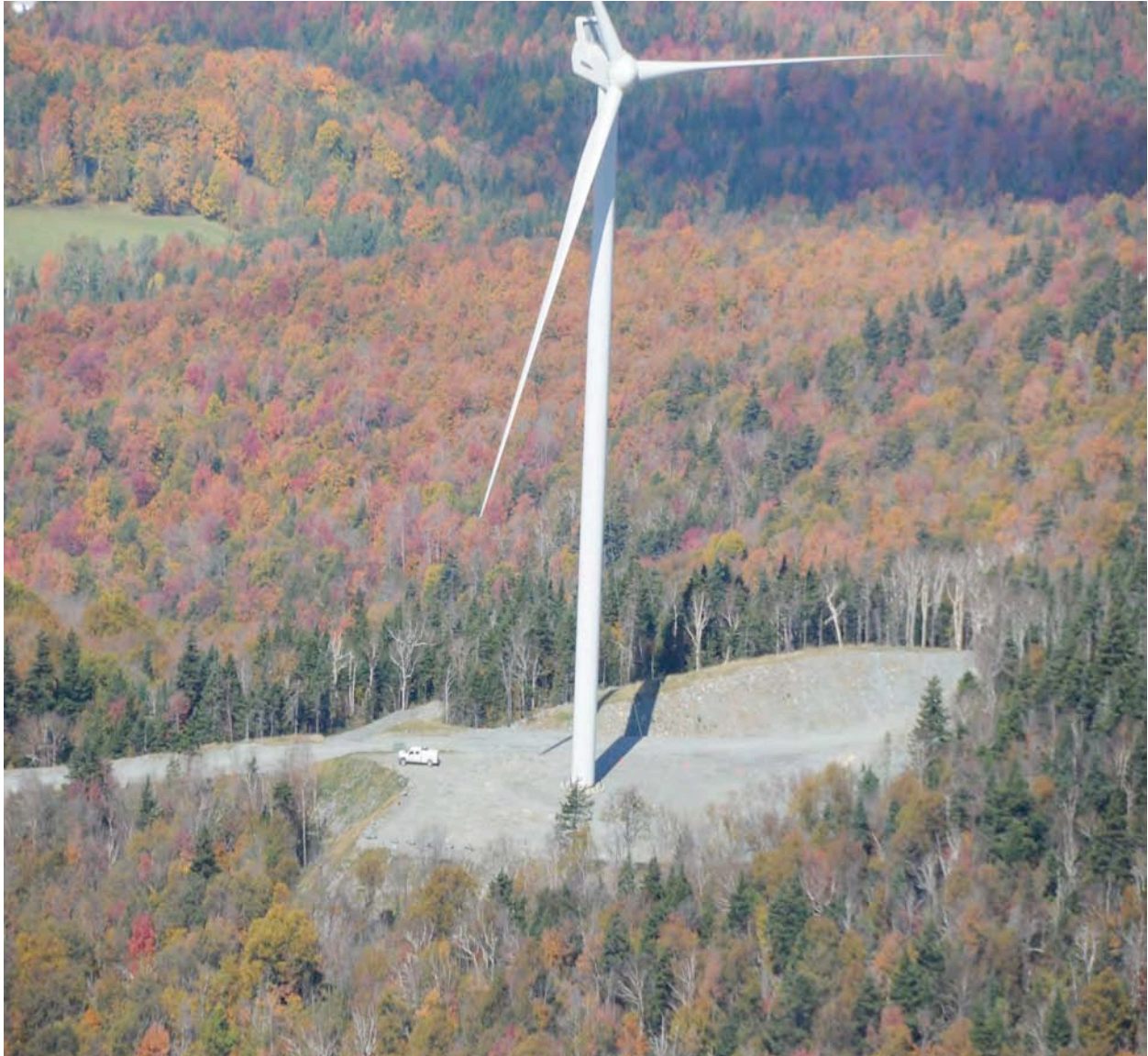
Tower Looming above Forest Floor, Lowell Mountain, Vermont Photo by Steve Wright
