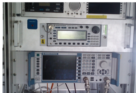
Rohde & Schwarz EVS 300 and EB200 installed in the ATR 42
