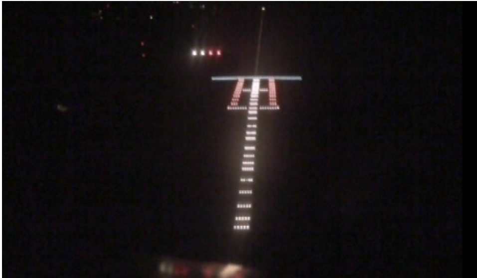
Figure 5. ALSF-2 As Re-configured on Runway 04 at KIAD
