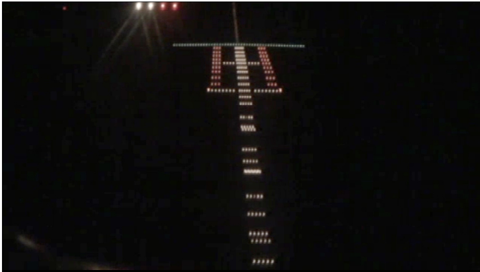
Figure 2. ALSF-2 As Installed on Runway 04 at KIAD
