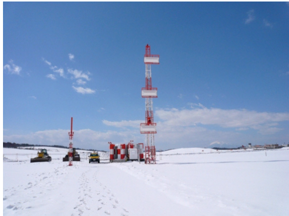
Fig 8.1: GS Antenna with Dual Frequency and 3 Elements in Snow Condition
