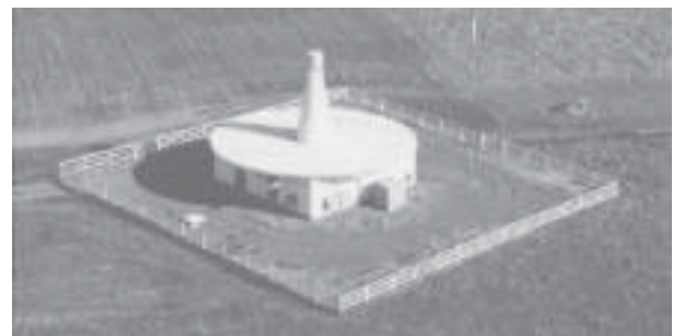
Figure 7. Circa 1950 – Early VOR ground equipment installation (from FAA archives)
