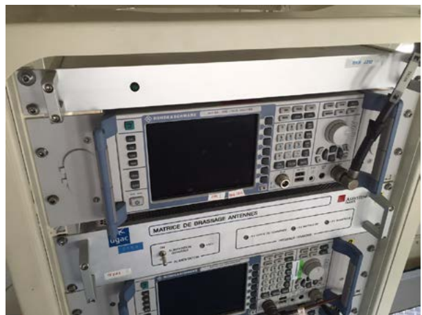
Figure 5. R&S@EDS300 Installation in the FI Aircraft
