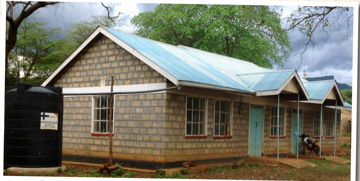
Barwessa Health Clinic, Baringo County - Hospital Staff Quarters
