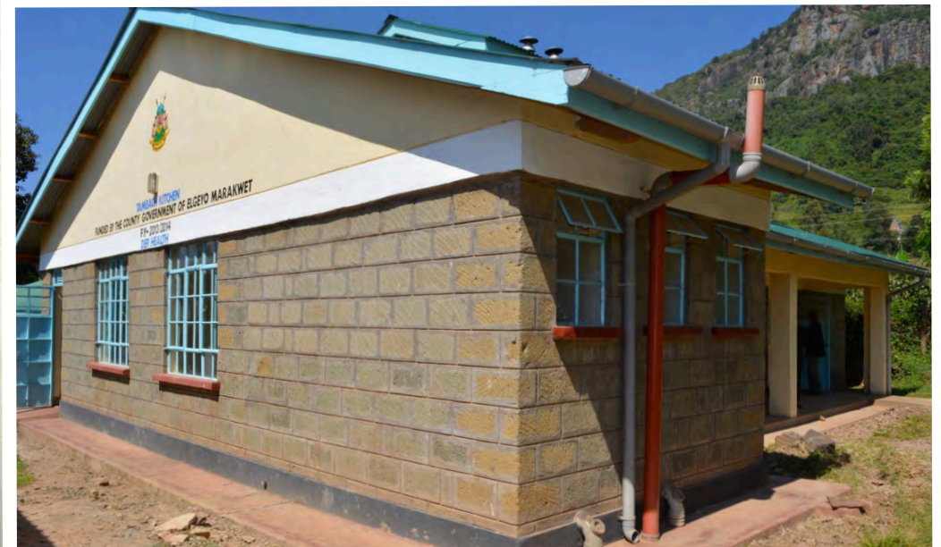
A new kitchen built in Tambach High School, Elgeyo Marakwet County
