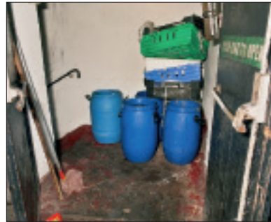
Figure 9: A blocked corridor
