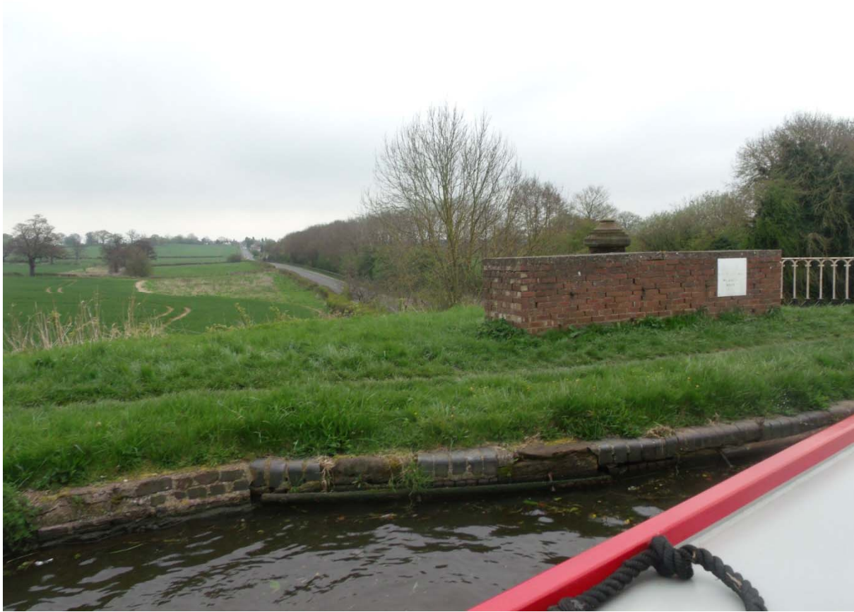
Stretton Aqueduct and the A5 or Watling Street
