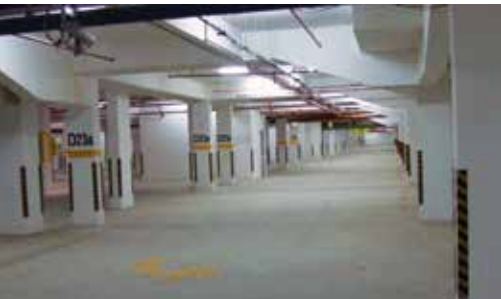
KK Times Square Underground Parking Kota Kinabalu, Malaysia
