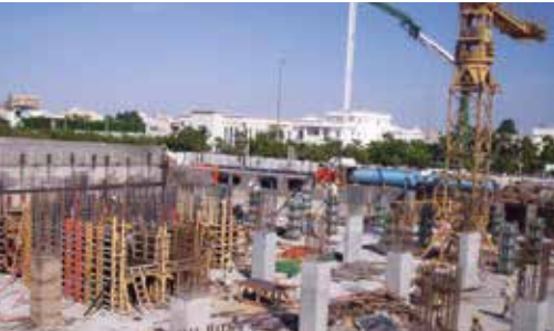
Al Mashfa Private Hospital Underground Parking, Jeddah, Saudi Arabia
