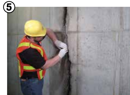
5 Waterproof leaking cracks and joints using the Krystol Leak Repair System.
