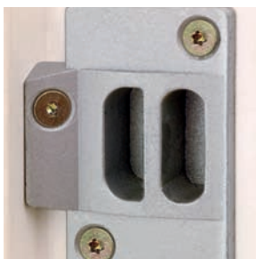
5. A security receiver with inclined screws fixed in the sturdy part of the frame makes it difficult to break open the window.
