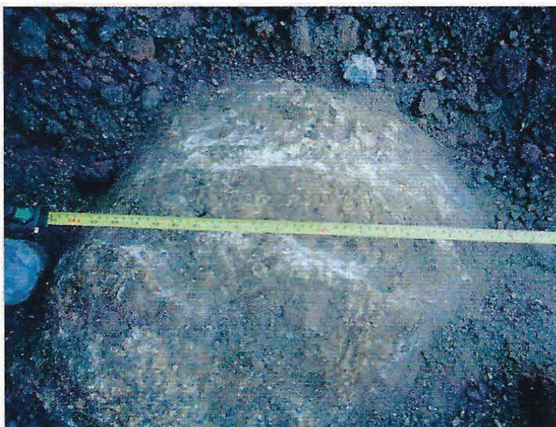
Single Rock Blasting
