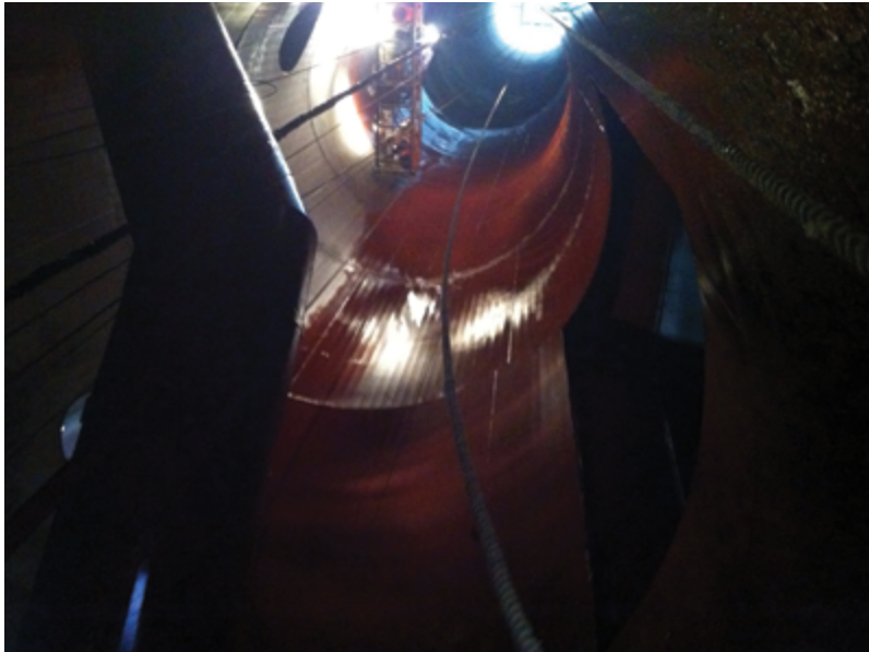
Corr-Paint™ CP2050-LF coats flare stack.
