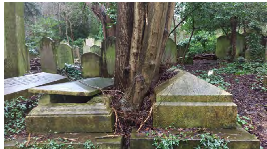
Fig. 79: A multi-stemmed elm growing between two tombs and causing damage in West Cemetery
