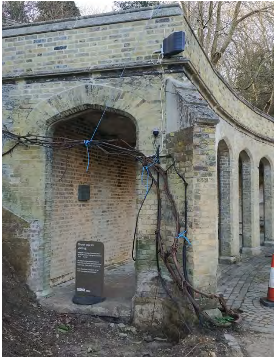
Fig. 111: Investigation works (March 2018) revealing original height of Colonnade plinth
