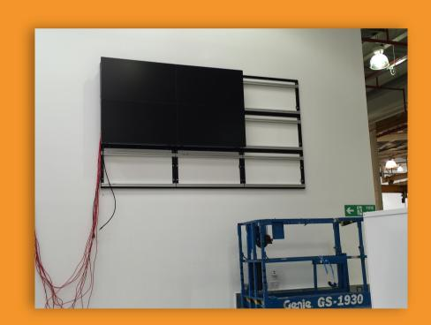
Top Left: Installing the framework using a MEWP
