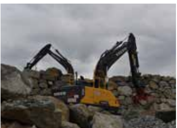
Used machinery; Machinery renovation (page. 4-5)
