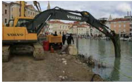
Underwater digging - Arm extension enables digging in positions that are much below excavator level - for example digging in the water (sea, river ...)
