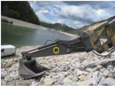
Long reach arm, an excellent, effective tool on site
