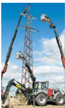
Kronos crane and working platform for lifting people
