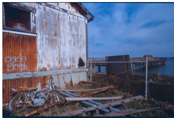
The rusty metal buildings, the debris—even this abandoned motorcycle—will be cleared away next month to make room for the Northwest Maritime Center.
