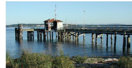
The 1930s-era dock at the Northwest Maritime Center is scheduled to be rebuilt this fall.
