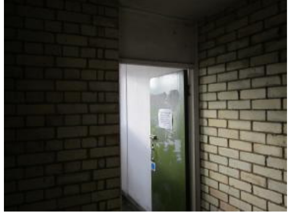
Chute room fanlights
