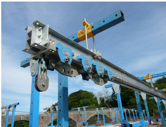
ADT and trolleys in place
