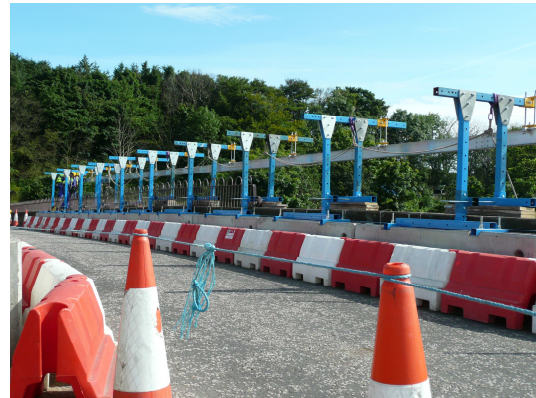
2 x 30M of ADST track & support blocks in place.
