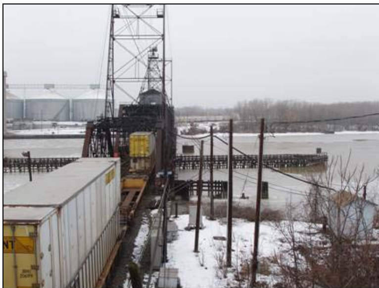
Photo 169: NS Maumee River Bridge, MP 287.6 – View West
