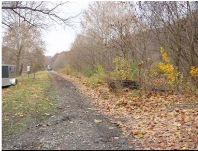
Photo 53: West end of POC track Walker's Mill MP 14.4
