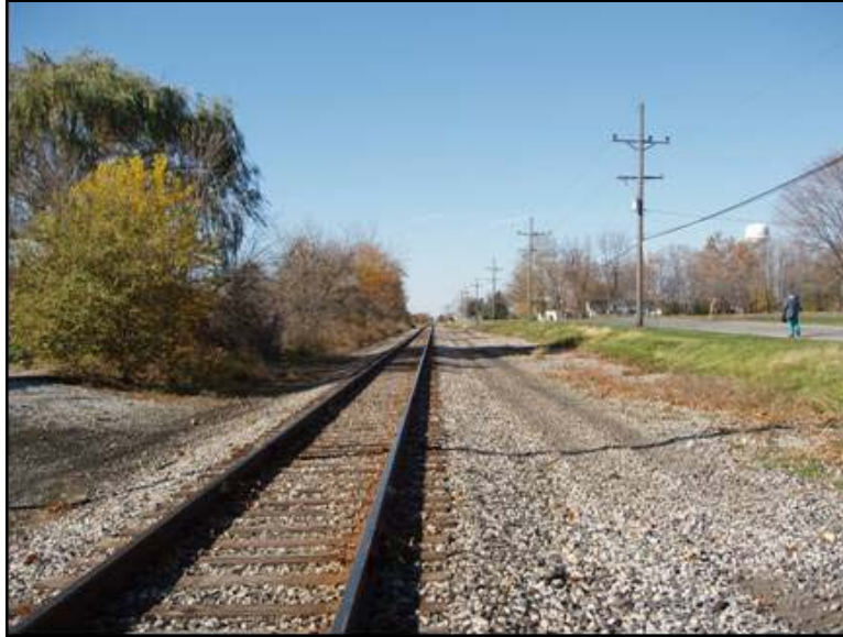
Photo 140: Fort Wayne Line, Washington St in Monroeville MP 304.3 – View west
