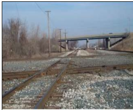
Photo 19: Looking north along CSX at Alexis Junction, CSX MP 57.7
