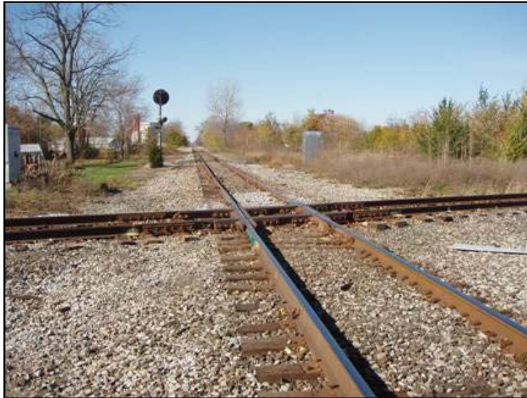
Photo 136: Fort Wayne Line, Diamond Crossing at Van Wert MP 287.7 – View west
