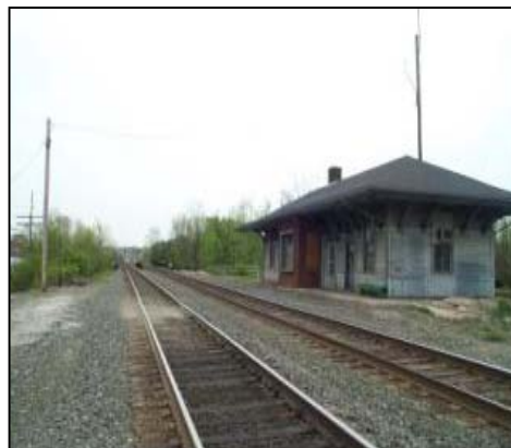
Photo 6: Looking south near Brown Street, NS MP 98 in Hudson
