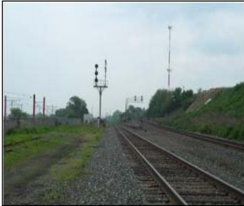
Photo 1: Looking east at CP 181 along CSX to Buffalo (left) and NS to Ravenna (right), just east of Cleveland Station
