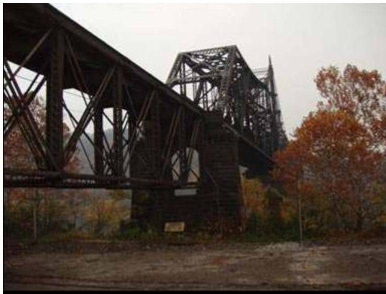
Photo 75: W&LE Bridge at Mingo Jct.
