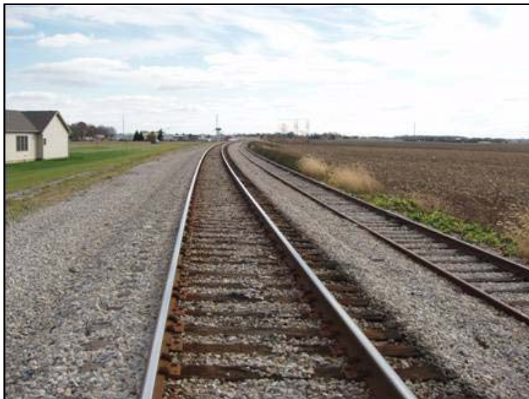
Photo 127: Fort Wayne Line east of Delphos MP 274 - View east
