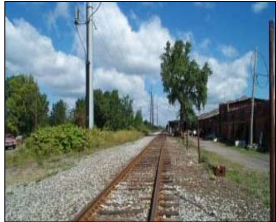
Photo 41: Looking north at CSX track at Scajaquada Creek, CSX MP 4.2
