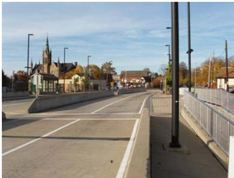
Photo 56: PAT West Busway, Crafton Station at PRR MP 6.0
