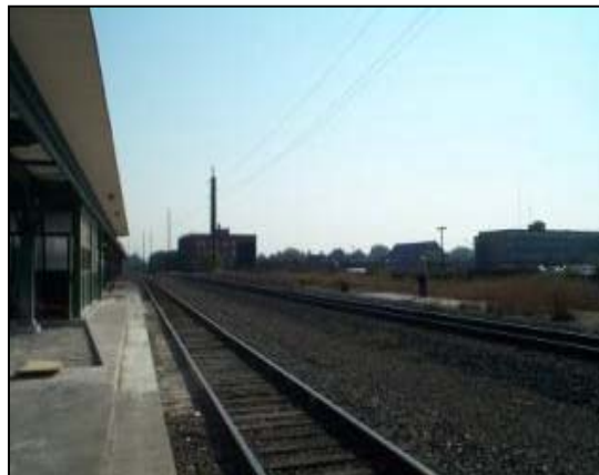
Photo 32: Erie Station, looking east
