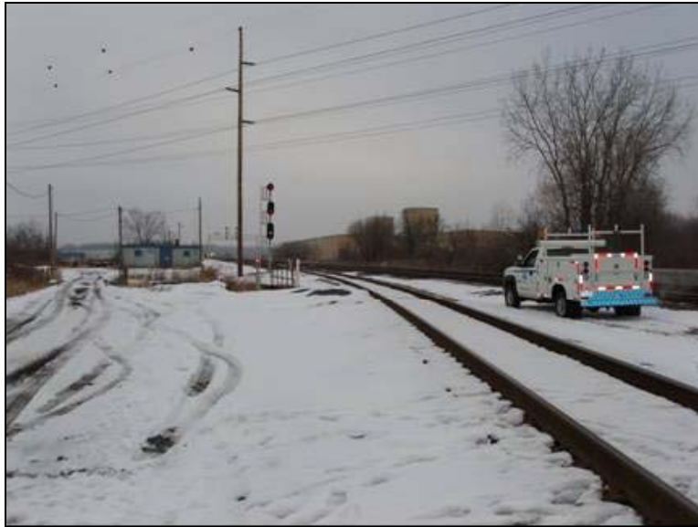
Photo 160: CSX Walbridge Junction CTT MP 20.8 – View West
