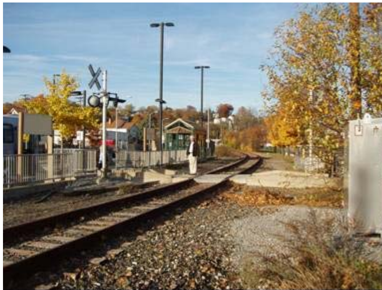
Photo 58: PAT West Busway, Carnegie Station at PRR MP 8.6
