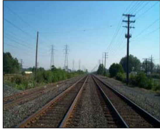
Photo 25: Looking east along CSX tracks at 305th Street, CSX MP 166.78
