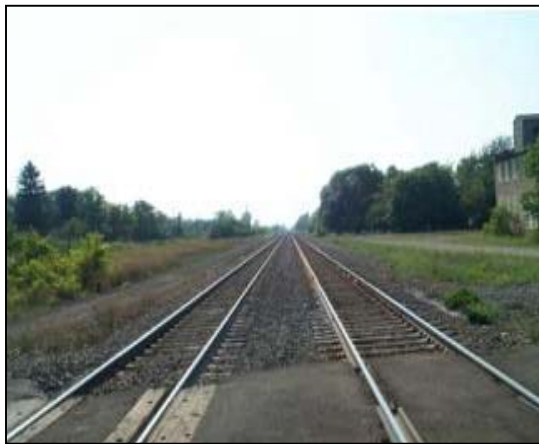
Photo 36: Looking east along CSX tracks at State St. in Ripley, CSX MP 65.3
