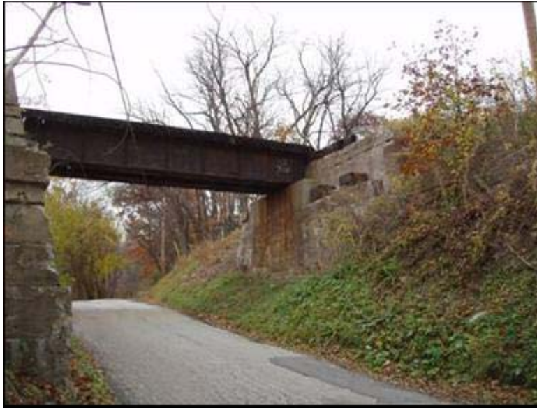
Photo 72: W&LE Bridge at Vienna, PA
