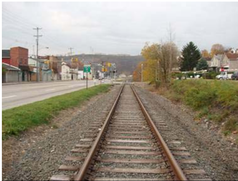
Photo 51: POC at Boyd Street in Carnegie, PA
