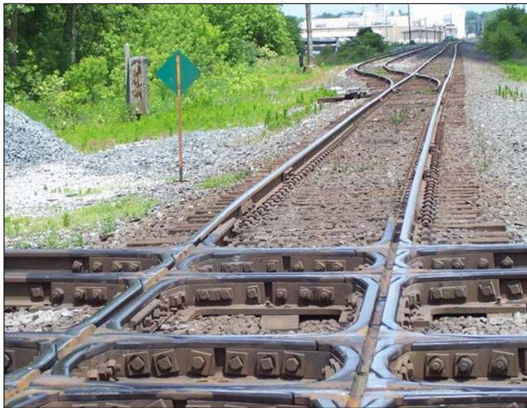
Photo 149: CSX Mainline Crossing at Galatea, OH – View North along Toledo Branch
