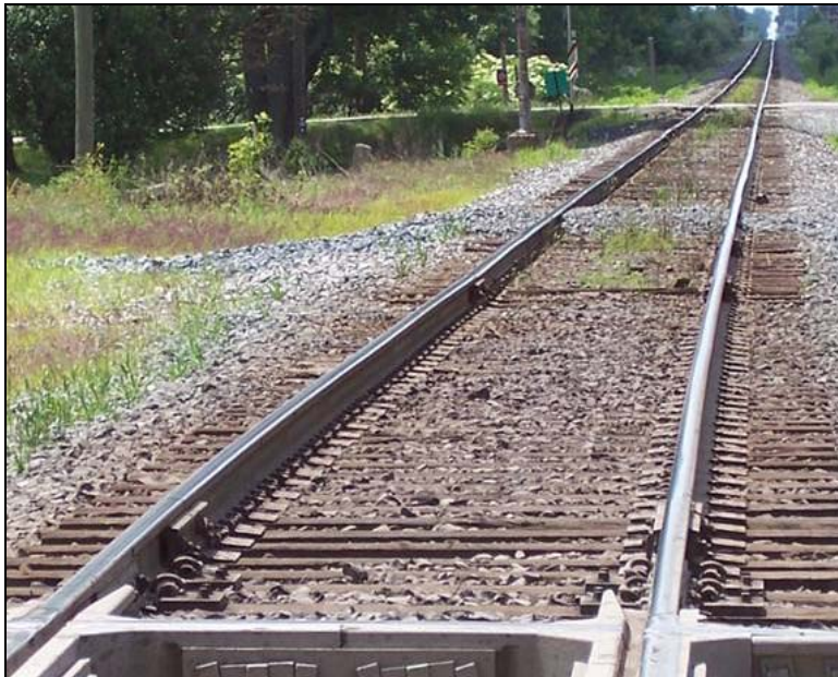
Photo 146: NS Mainline Crossing at Mortimer, OH – View South
