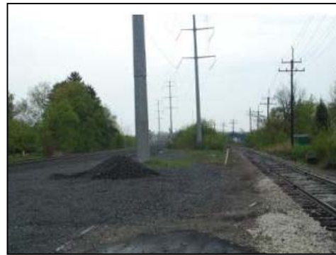
Photo 4: Looking north at Glendale Road, NS MP 110. NS tracks are on left, W&LE on right. A connection would be made in this area from the NS corridor to the W&LE tracks.
