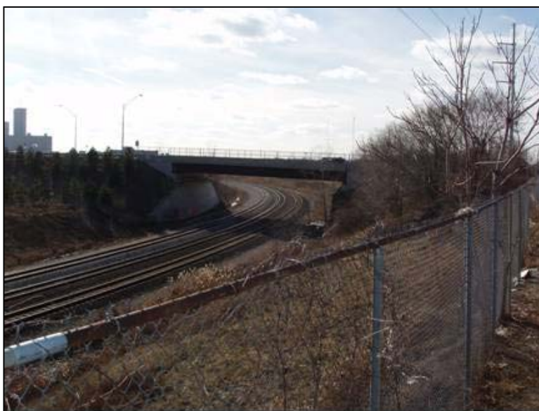
Photo 96: Columbus, OH, C&N MP 136.1 – Cleveland Ave Overpass – View West
