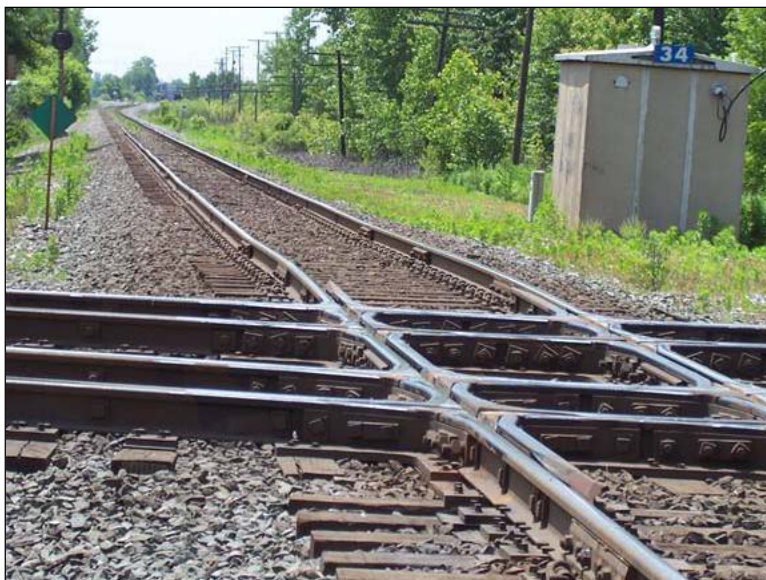
Photo 147: CSX Mainline Crossing at Galatea, OH – View South along Toledo Branch
