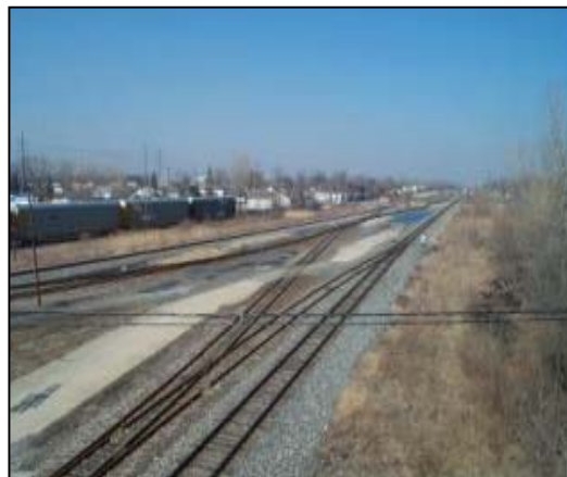
Photo 18: Looking north at CN MP 36.6, from West Road overpass
