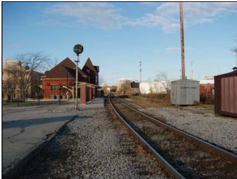
Photo 125: Fort Wayne Line at Lima crossing CSX/NS MP 260.3 - View west
