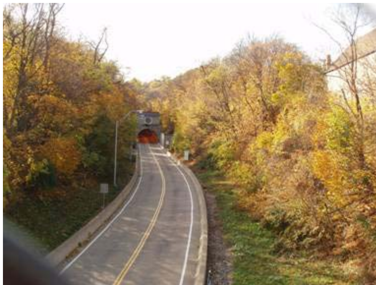
Photo 54: PAT West Busway, Corliss Tunnel portal at PRR MP 4.7
