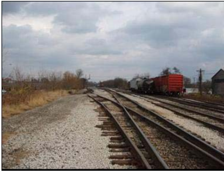
Photo 95: Newark, OH, C&N Subdivision MP 104.6 – View West
