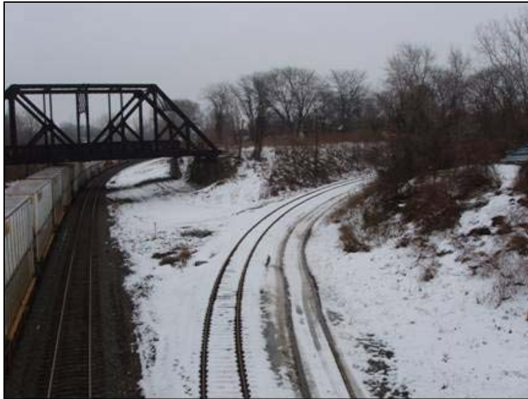
Photo 168: Miami Cut branch diverging from the NS Cleveland-Chicago Mainline MP 287.5 – View east
