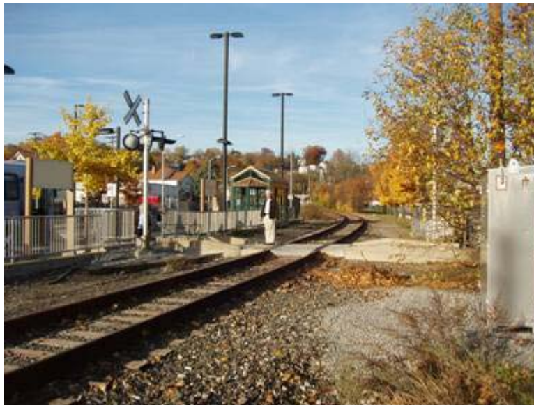
Photo 50: POC Railroad (former PRR Panhandle) at Carnegie, with adjacent PAT busway
