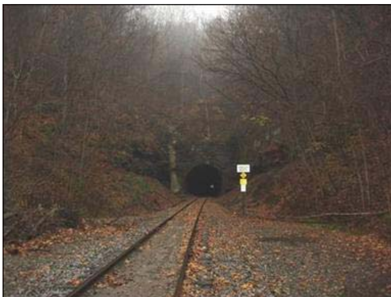
Photo 77: East Portal, Gould Tunnel
