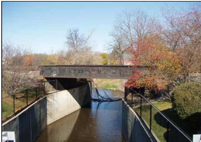
Photo 135: Fort Wayne Line, Town Creek bridge at Van Wert MP 287.6
