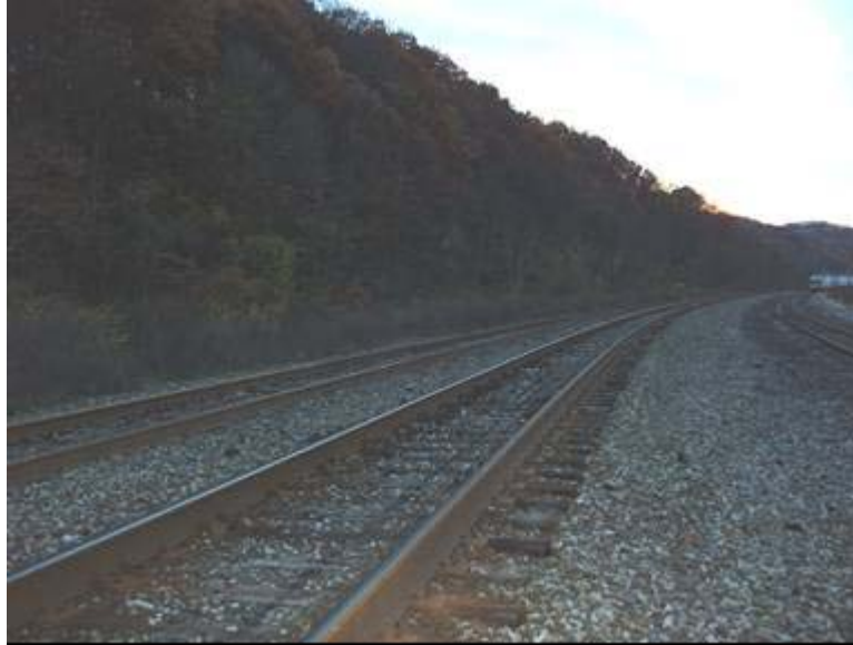
Photo 49: POC Railroad double track south (railroad west) of Duff's Junction
