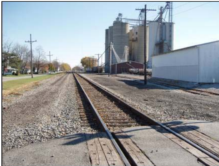
Photo 141: Fort Wayne Line, Washington St in Monroeville MP 304.3 – View east
