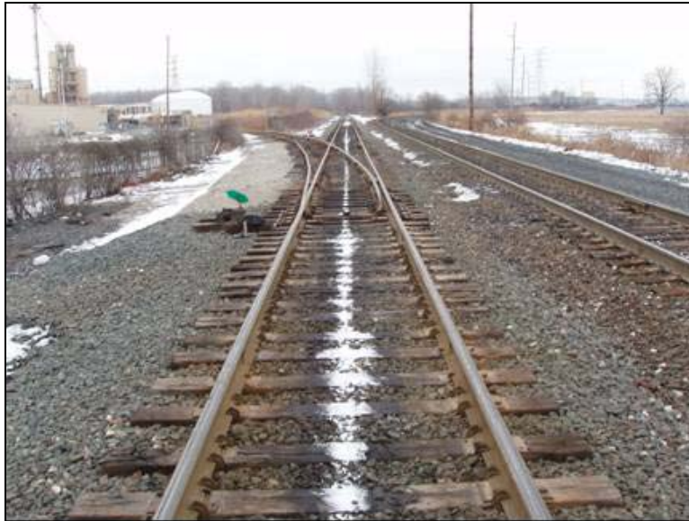
Photo 152: CSX Toledo Branch, Tracy Road Crossing – View East
