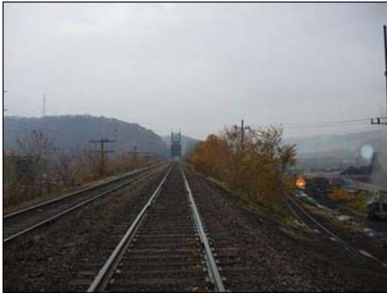
Photo 74: W&LE Bridge at Mingo Jct.
