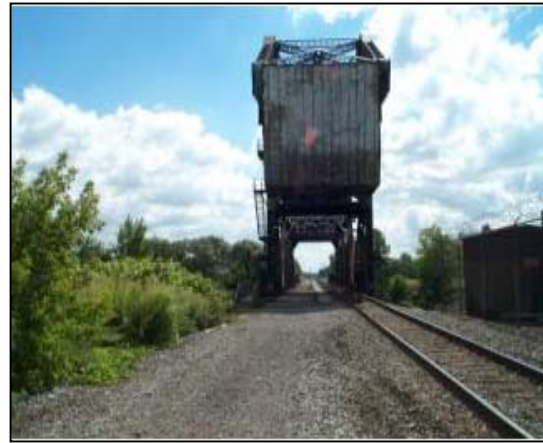
Photo 39: Looking south over the Buffalo River Bridge
