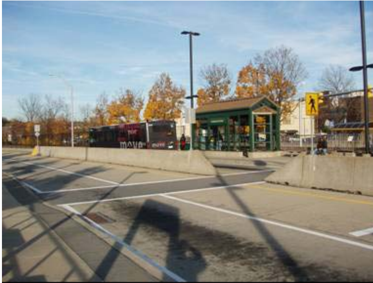
Photo 57: PAT West Busway, Carnegie Station at PRR MP 8.6
