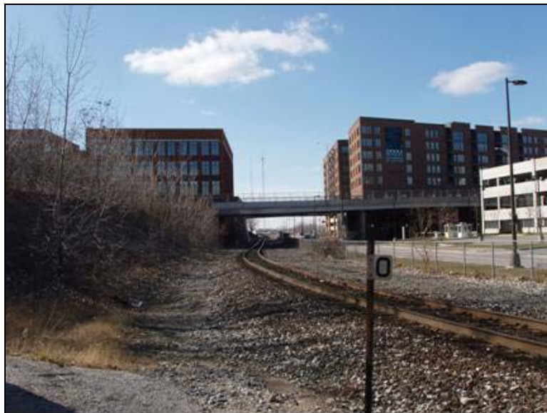
Photo 102: Columbus, OH, Buckeye Line West of CP-138 – View West from High Street towards Front Street
