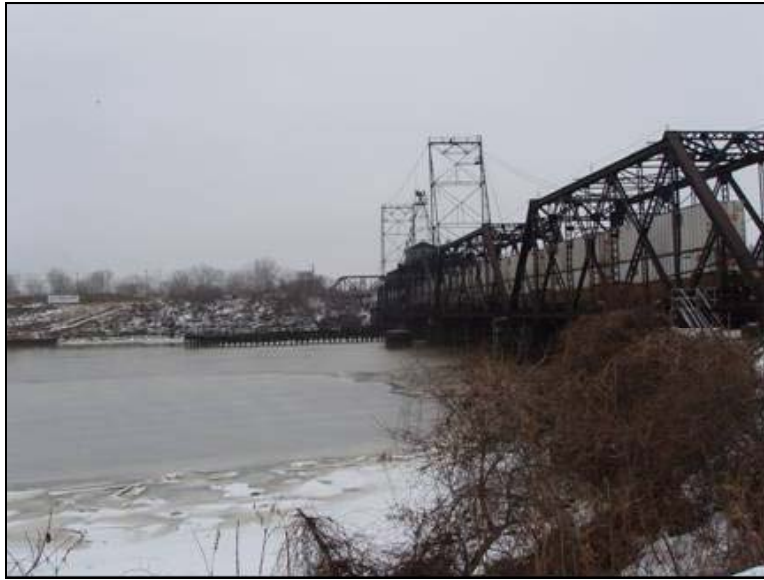
Photo 170: NS Maumee River Bridge, MP 287.6 – View East
