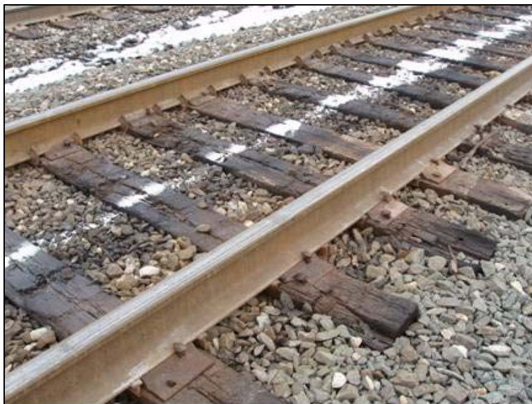
Photo 153: CSX Toledo Branch, Tracy Road Crossing – Close up of Track
