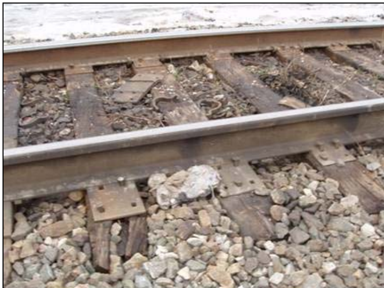
Photo 157: CSX Toledo Terminal, Broadway Road Crossing – Close up of Track
