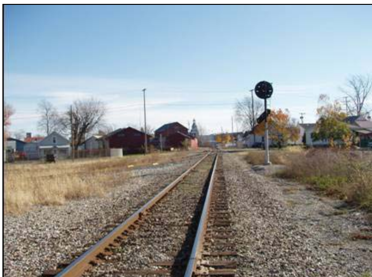
Photo 137: Fort Wayne Line, Diamond Crossing at Van Wert MP 287.7 – View east
