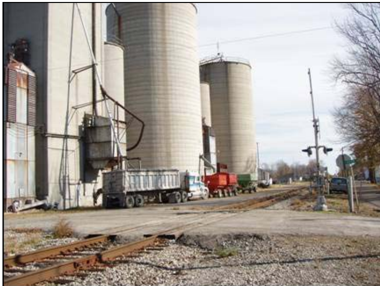
Photo 131: Fort Wayne Line, Mason St grade crossing MP 280.3 in Middlepoint - View east
