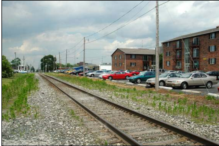
Photo 150: CSX Toledo Branch, Bowling Green, OH – View North
