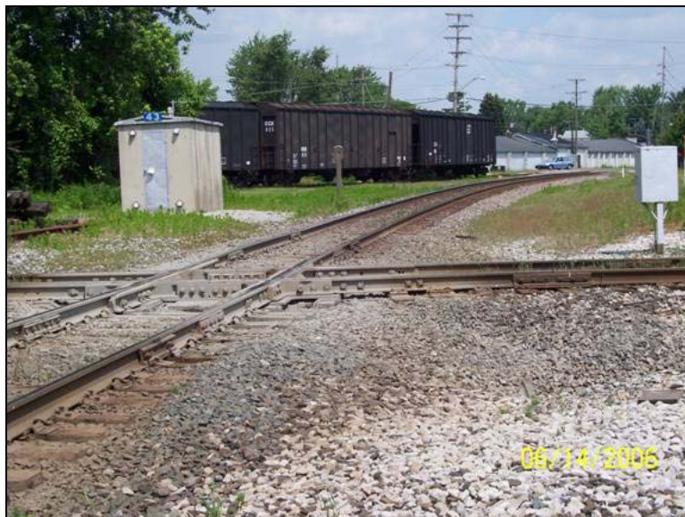
Photo 143: NS Lima Branch crossing at Findlay, OH – View North
