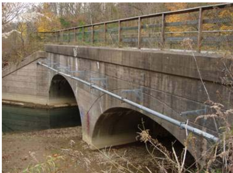
Photo 60: Panhandle Bridge over Chartier's Creek – Downstream View
