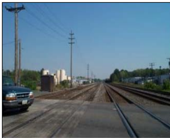
Photo 27: Looking east along CSX at Newell Street, CSX MP 154.68
