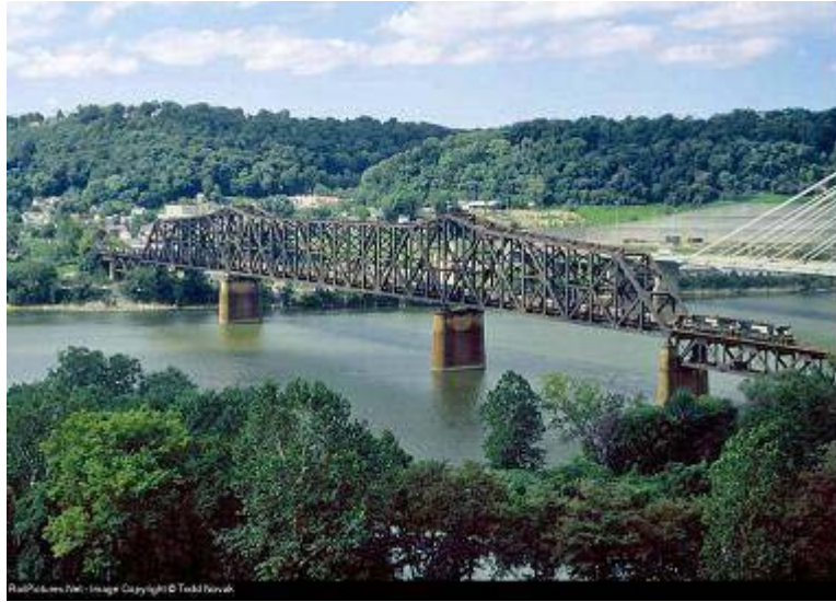
Photo 65: PRR Panhandle Bridge at Weirton. © Todd Novak, Used with Permission
