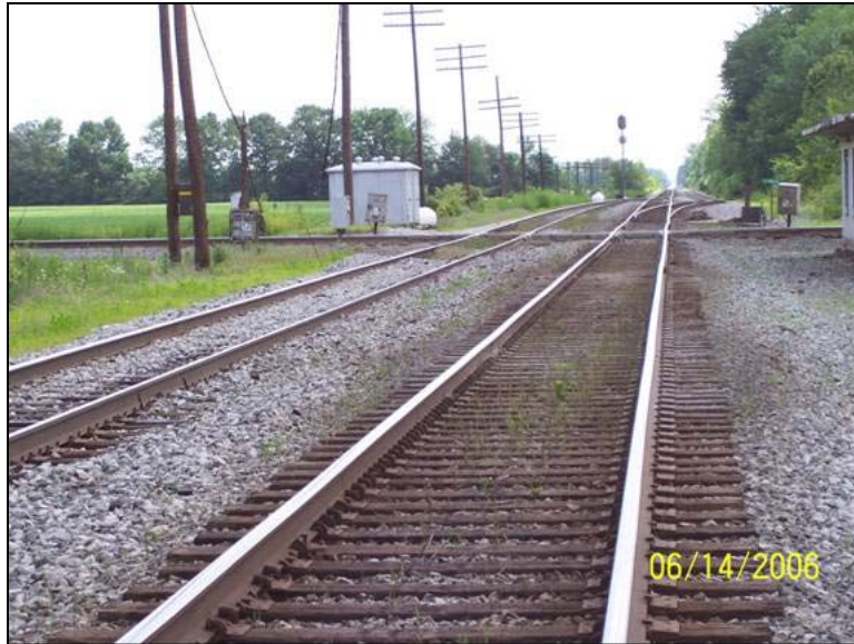
Photo 144: NS Mainline Crossing at Mortimer, OH – View East
