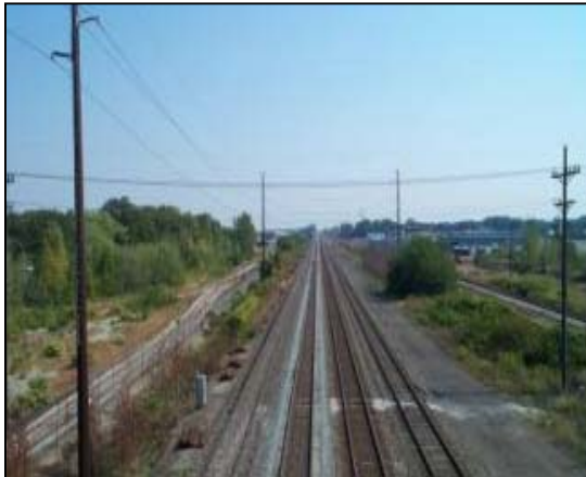
Photo 34: CSX MP 84 at Franklin Ave., looking east. The tracks on the left are the GE plant testing tracks also used to connect to the CSX mainline.
