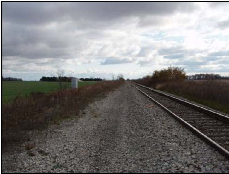
Photo 118: Fort Wayne Line at Dola, MP 238 - View east
