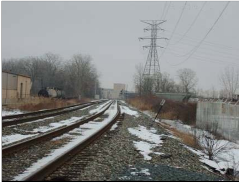
Photo 154: CSX Toledo Terminal, MP 19.0 – View East
