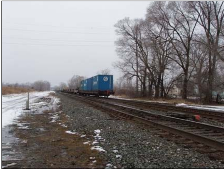
Photo 166: Norfolk Southern Cleveland-Chicago Mainline at CP 286 - View west
