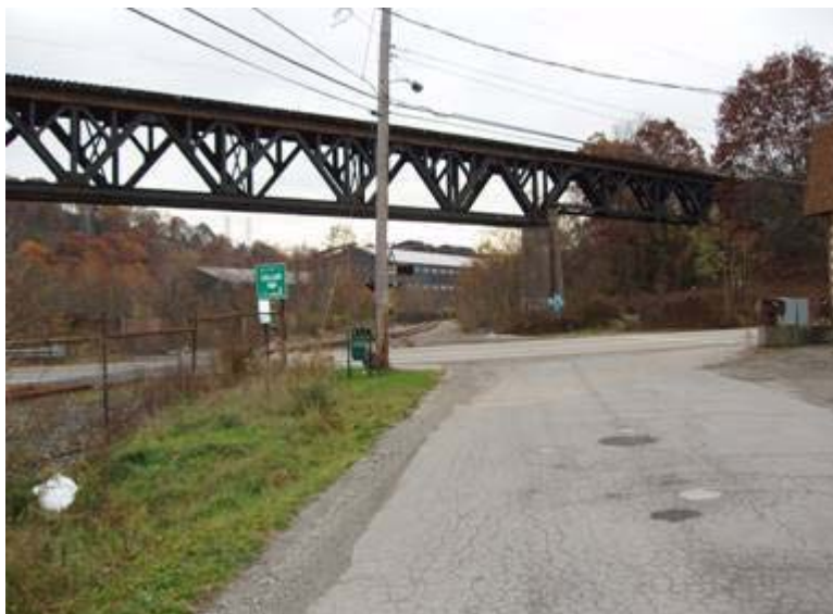
Photo 71: W&LE and PCY Crossing, View West
