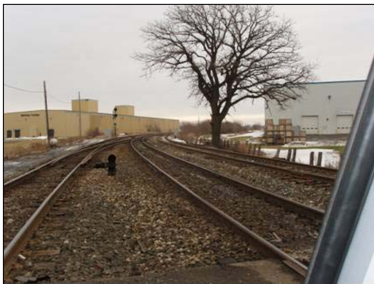
Photo 155: CSX Toledo Terminal, Broadway Road Crossing – View East
