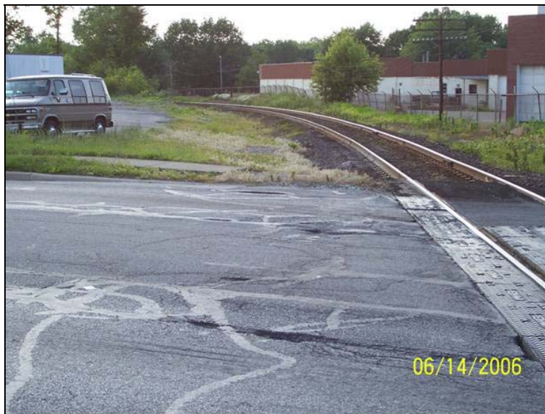
Photo 105: CSX Scottslawn Subdivision, Delaware Ave at Marysville – View North
