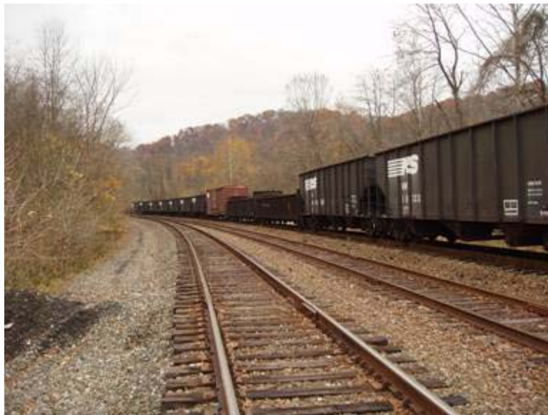
Photo 66: NS/OHCR Interchange Track East of Gould Tunnel
