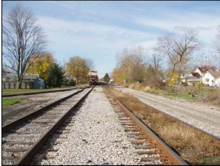
Photo 130: Fort Wayne Line west of Delphos MP 275 - View west
