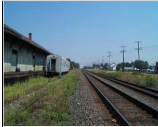
Photo 35: At Northeast station looking east along CSX tracks, CSX MP 72
