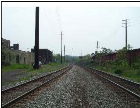
Photo 3: Looking south along the NS Cleveland Line at MP 118.5
