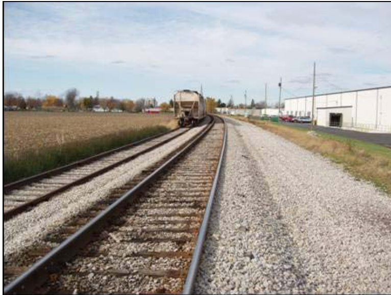
Photo 126: Fort Wayne Line east of Delphos MP 274 - View west
