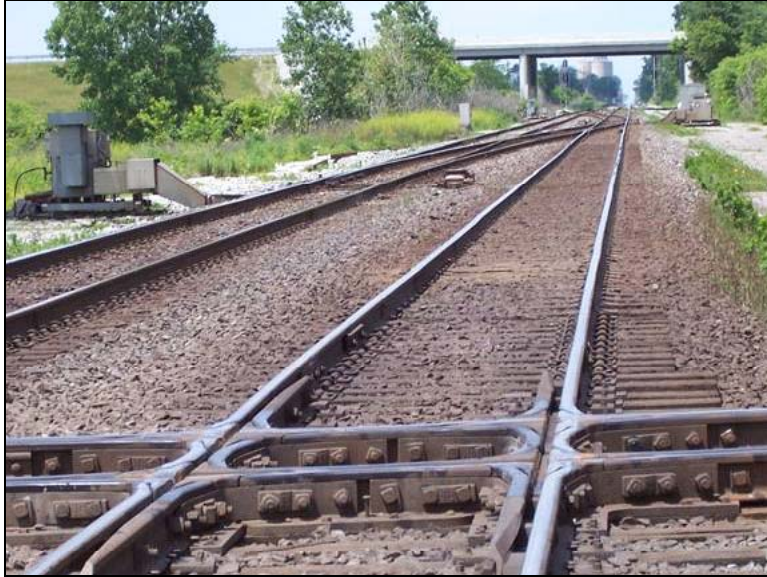
Photo 148: CSX Mainline Crossing at Galatea, OH – View West along CSX Mainline
