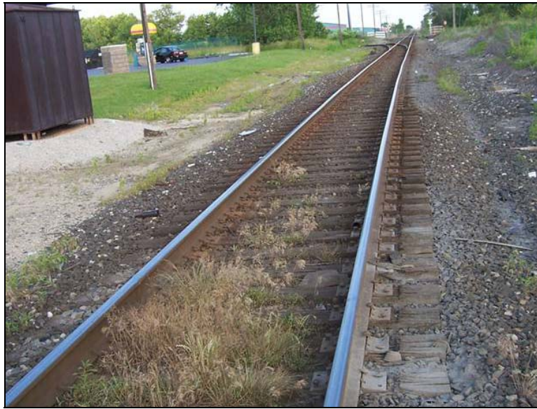
Photo 104: CSX Scottslawn Subdivision, Delaware Ave at Marysville – View South
