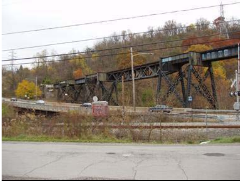
Photo 70: W&LE and PCY Crossing, View East
