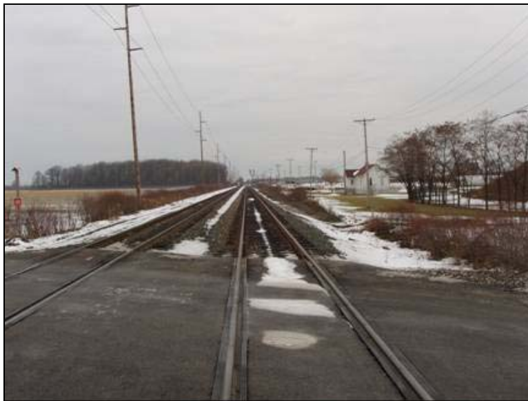
Photo 151: CSX Toledo Branch, Tracy Road Crossing – View West
