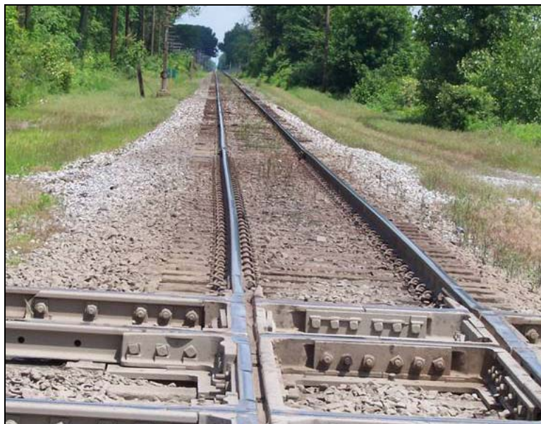
Photo 145: NS Mainline Crossing at Mortimer, OH – View North
