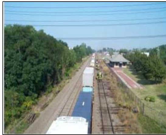
Photo 37: Looking east along CSX from SR 394 overpass, CSX MP 57.54
