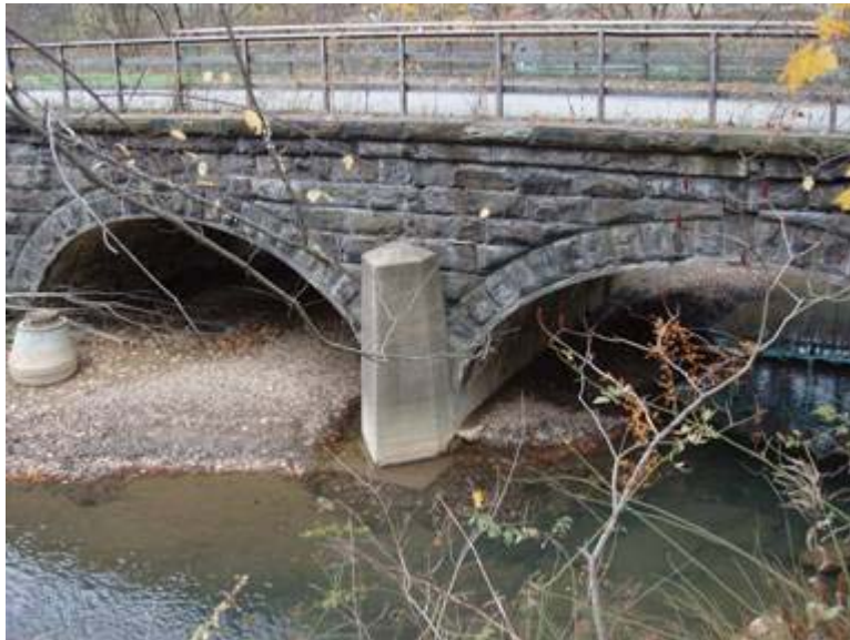
Photo 61: Panhandle Bridge over Chartier's Creek – Upstream View
