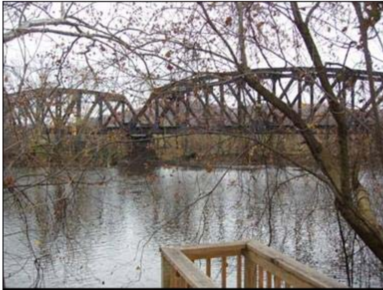
Photo 84: Muskingum River Bridge
