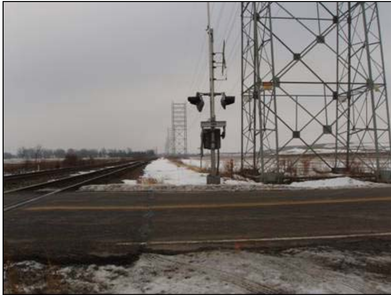
Photo 162: CSX Toledo Terminal, Wales Road Crossing CTT MP 21.7 – View South
