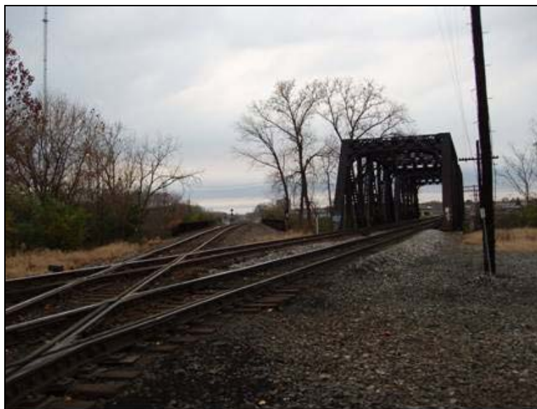
Photo 103: CP Hocking view west along the Buckeye Line. The double-tracked CSXT line to Marion passes through the girder bridge on the right.
