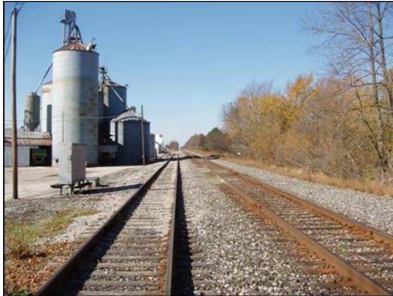
Photo 138: Fort Wayne Line, Convoy MP 294.7 – View west
