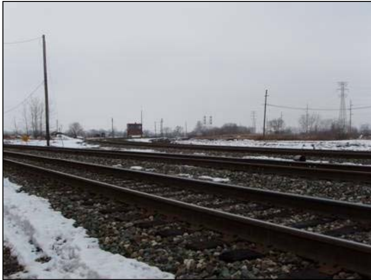
Photo 158: CSX Toledo Terminal CTT MP 20.8, Walbridge Interlocking
