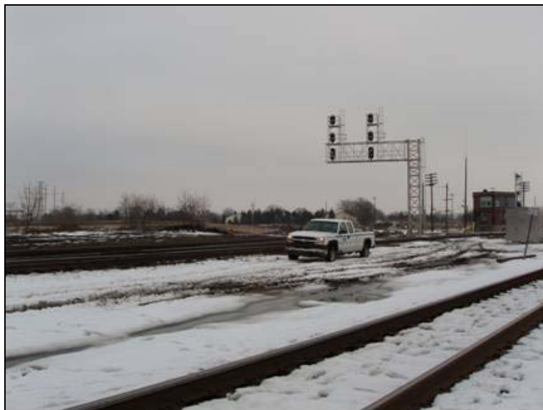
Photo 159: CSX Walbridge Junction CTT MP 20.8 – View East
