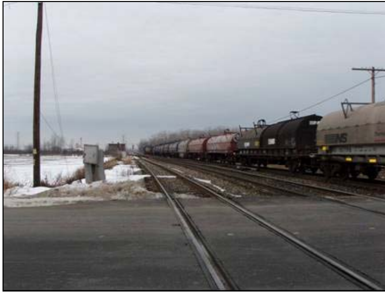
Photo 156: CSX Toledo Terminal, Broadway Road Crossing – View West
