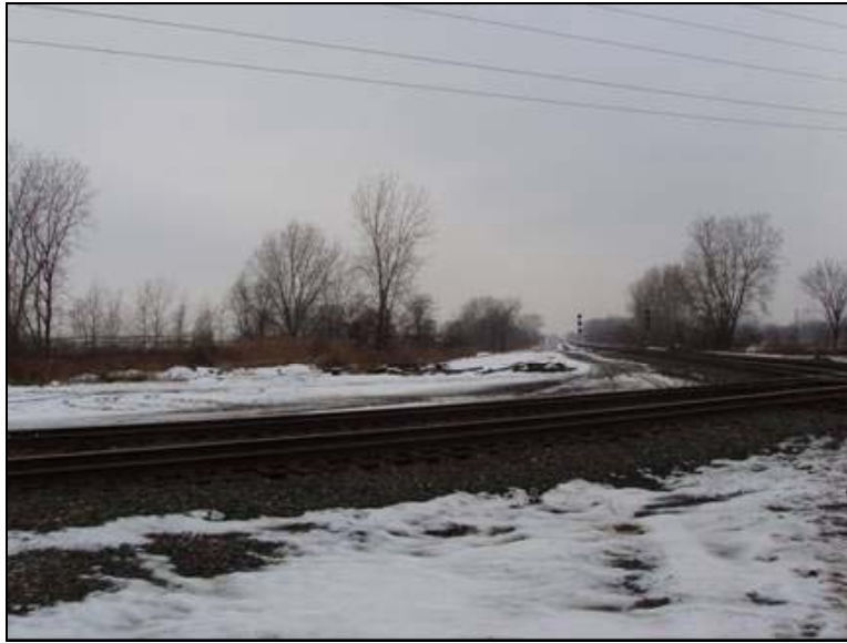
Photo 164: CSX – NS Junction at Vickers – View across Southwest Quadrant, West towards Toledo
