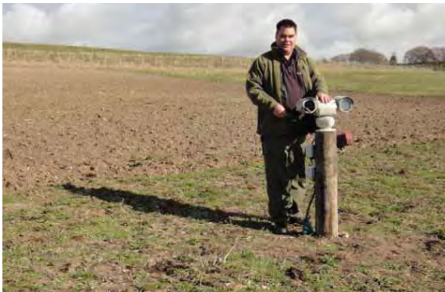
Charles set up the CCTV cameras at the Project Site after quite a learning curve!
