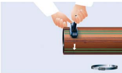
Fig 8-34: Removal of the protective coating with the egeplast M10 peeling tool
