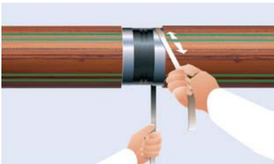
Fig 8-39: Rubbing down the aluminium foil
