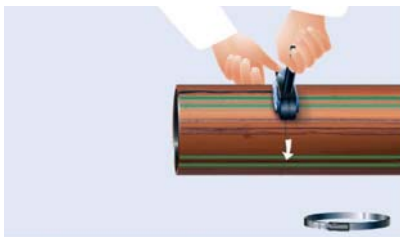
Fig 8-18: Removal of the protective coating with the egeplast M10 peeling tool
