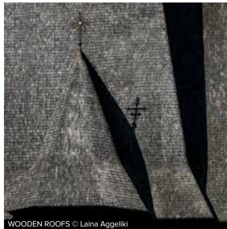
WOODEN ROOFS © Laina Aggeliki
