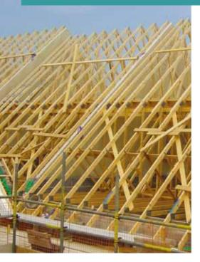
Spandrel panels are specially designed and factory-produced timber framed panels to construct separating walls, that would otherwise have to be constructed throughout in masonry.
