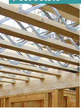
Posi-Joists<sup>™</sup> allow building designers the freedom to have a variety of internal room layouts without the constraints of solid and other engineered timber joists.
