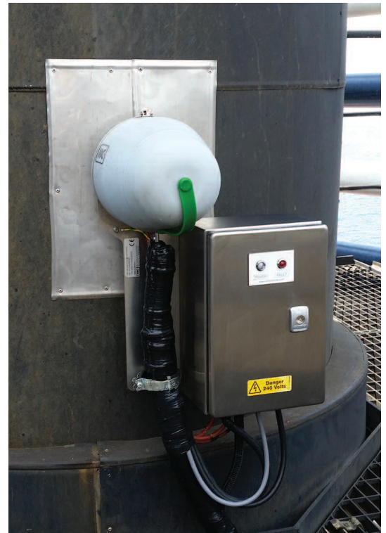
Emsys probes are powered from the main enclosure meaning only a single power supply is required
