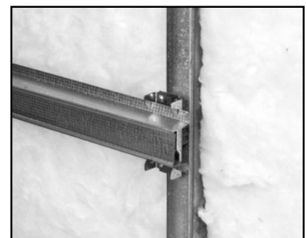
Figure 2.2: Snap hat channel into clip
