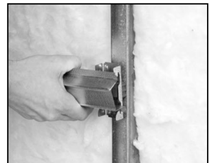
Figure 2.2: Snap hat channel into clip
