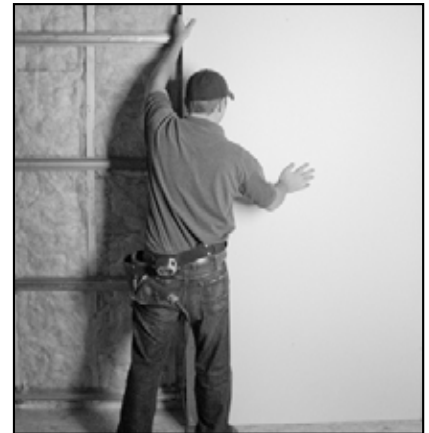
Figure 3.2: Install drywall vertically to hat channels
