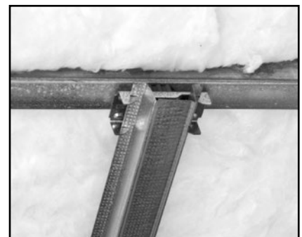
Figure 5.2: Snap Hat Channel into Clip
