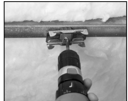
Figure 5.1: Screw A237R into joists
