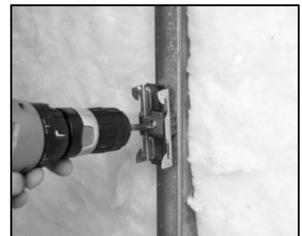
Figure 2.1: Screw clips into stud wall
