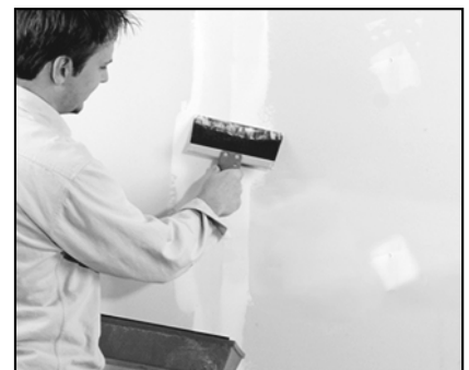
Figure 3.4: Tape and mud drywall
